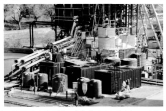
Figure A3.4. The Rhodes BioSURE Process<sup>®</sup> pilot plant constructed in Grahamstown by Grahamstown Engineering Co., transported to Grootvlei Gold Mine, Gauteng, and erected on site.
