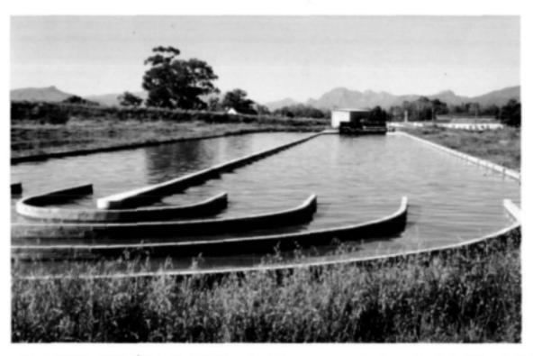
Figure 5.4. The 2500 m<sup>2</sup> Spirulina-HRAP constructed as a component unit operation in the full-scale IAPS treating tannery wastewaters at Mossop-Western Leathers Co., Wellington.
