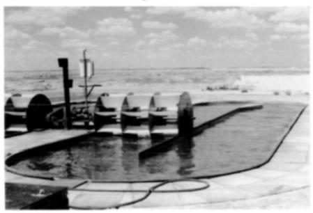
Figure 4. The pilot-scale *Dunaliella*-HRAP developed for the treatment of organic contamination in saline carbonate brines at the Botswana Ash Co. Sua Pan, Botswana.
