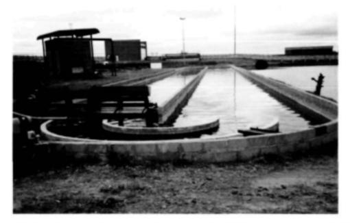
Figure 8.6. The High Rate Algal Pond unit operation of the IAPS plant constructed at the Cato Ridge Abattoir for the treatment of abattoir wastewaters.
