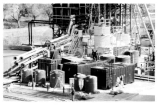
Figure 7. The Rhodes BioSURE<sup>\*</sup> pilot plant located at Grootvlei Mine, Gauteng Province, and using primary sewage sludge as the carbon source in the treatment of acid mine drainage wastewaters.
