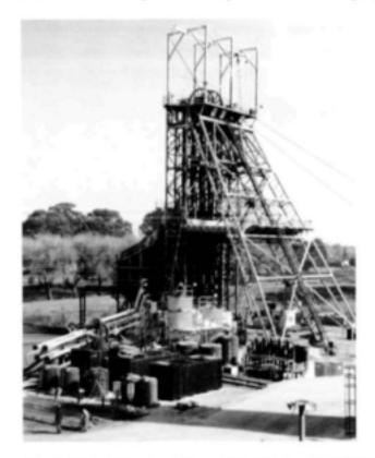
Figure 7.2. Headgear at the No.4 shaft Grootvlei Mine with the Rhodes BioSURE Process® pilot plant in the foreground. Reactors were constructed in Grahamstown, and then transferred to site.
