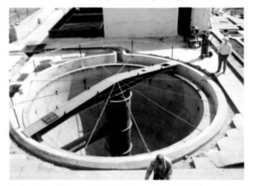
Figure 8. The scaled-up 2 ML Recycling Sludge Bed Reactor in the BioSURE<sup>®</sup> sewage sludge solubilisation technical-scale plant constructed at Erwat's Ancor Works in Springs. Surface struts provide support for a covering membrane.
