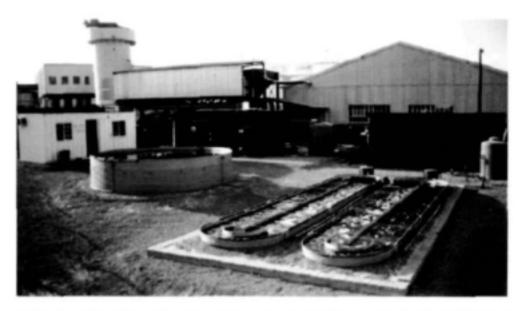
Figure 8.7. Pilot plant at Brennokem Co., in Worcester, South Africa, evaluating the IAPS in the treatment of wine lees and distillery wastewaters.
