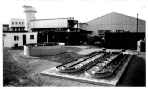
Figure 9. Integrated algal ponding system pilot plant constructed at the Brennokem Co. wine lees plant in Worcester, South Africa, for the treatment of winery, and saline distillery and wine lees wastewaters.
