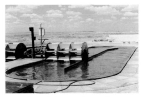
Figure 6.3. The Dunaliella-HRAP pilot plant treating saline carbonate brines at Botswana Ash Co., Sua Pan, Botswana.
