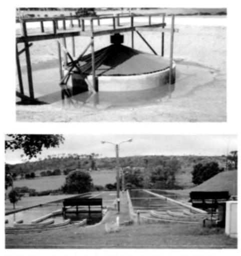
Figure 8.2. The Primary Facultative Pond and High Rate Algal Ponds of the AIWPS process constructed at the Grahamstown IAPS demonstration and research plant treating domestic wastewaters.
