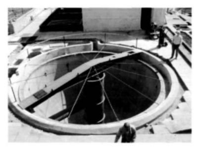
Figure 7.17. The 2 ML scaled-up Recycling Sludge Bed Reactor in the BioSURE<sup>®</sup> sewage sludge solubilisation technical-scale plant constructed at Erwat's Ancor Works in Springs. Surface struts provide supports for a covering membrane.
