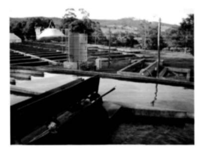
Figure 8.4. The Independent High Rate Algal Pond (I-HRAP) unit operation for tertiary treatment and the renovation of raw water at the Environmental Biotechnology Field Station, Grahamstown. The I-HRAP is in the foreground with the Algal Denitrification Bioreactor (ADB) column and the algal settling tank behind.
