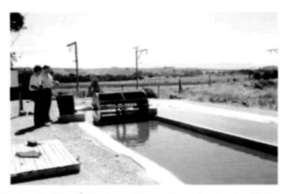
Figure 5.3. The Spirulina-HRAP pilot plant at Mossop-Western Leathers Co., Wellington, showing one of the 80 m<sup>2</sup> High Rate Algal Ponds.
