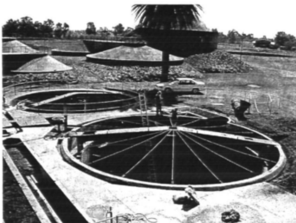
Figure A 4.2. The 2 ML scaled-up Recycling Sludge Bed Reactor in the BioSURE ® sewage sludge solubilisation technical-scale plant constructed at Erwat's Ancor Works in Springs. Surface struts provide supports for a covering membrane.
