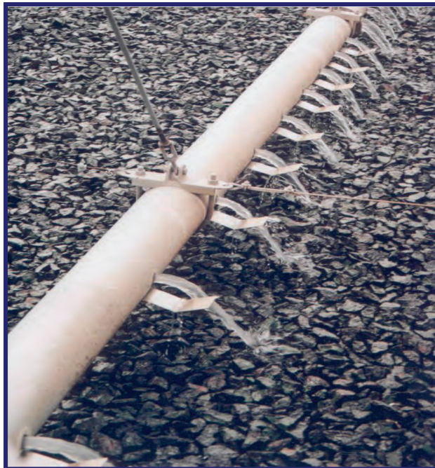
Figure 3.3 (g): Poor Splash Plate Design and Inadequate Feed Spreading
