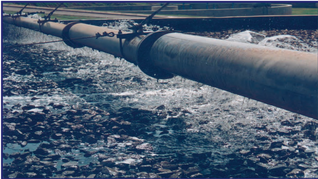
Figure 2.2 (a) : Ponding and Poor Drainage of the Filter
