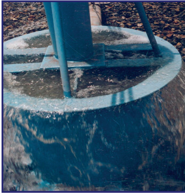
Figure 3.3 (f): Spilling Across the Centre Distribution Well
