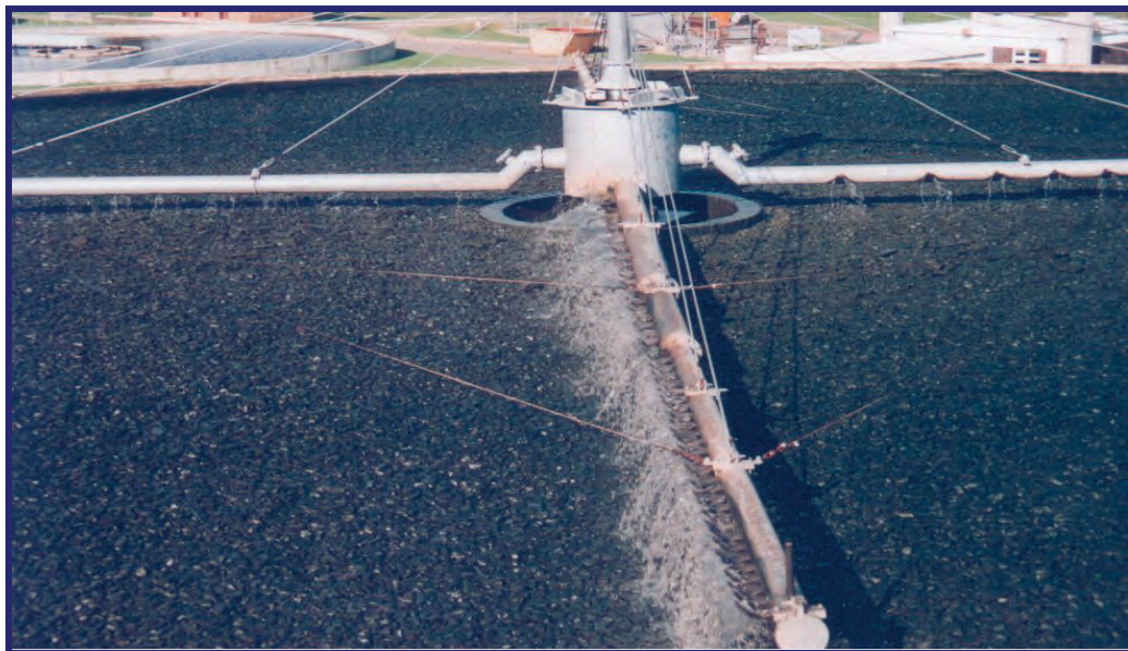
Figure 3.3 (i): Good Filter Feed Distribution Pays Dividends
