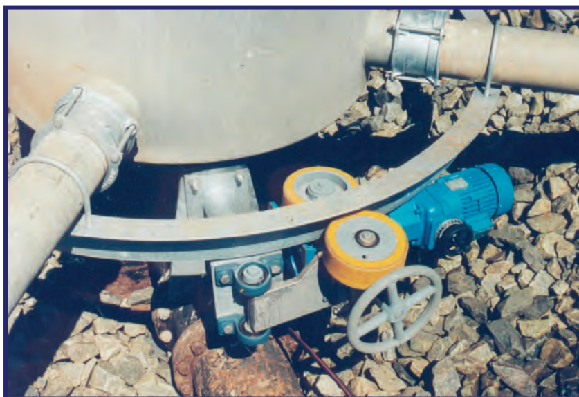
Figure 8.6 : Typical Centre Column Mechanical Drive Installation
