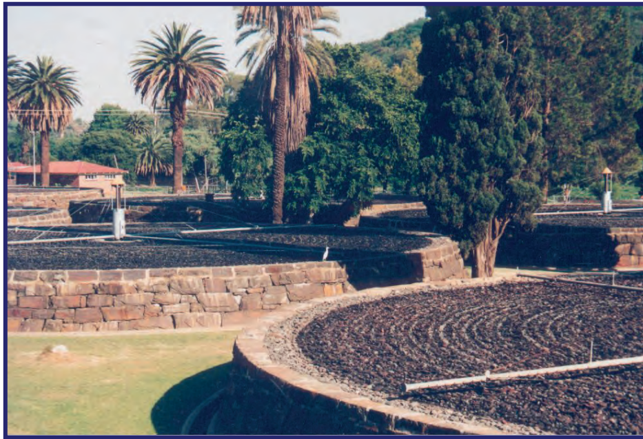
Figure 8.2 (a): Filter Walls Constructed of Cut Sandstone Blocks
