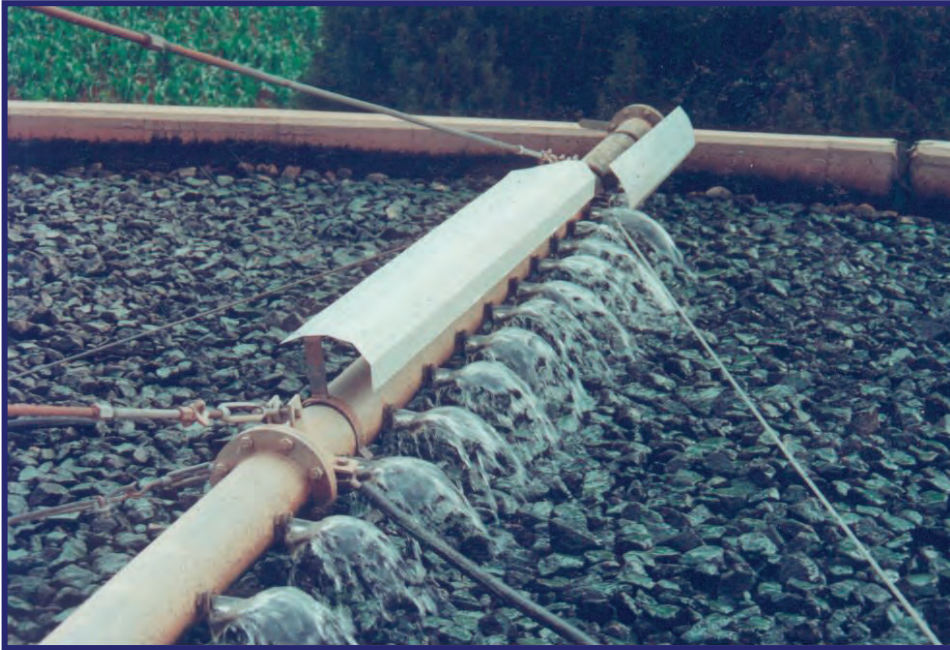
Figure 3.5 (b): Adjustable Braker Plates
