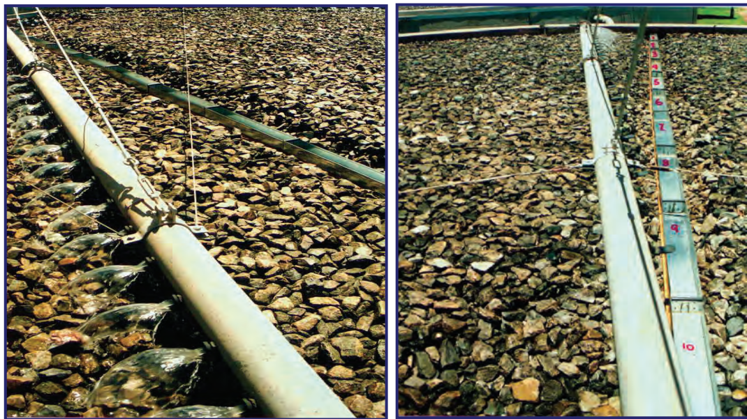
Figure 3.3 (c): Radial Troughs Across the Filter Media
