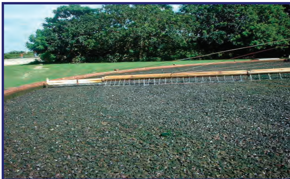
Figure 3.5 (c): Verulam Trickling Filters with Installed Breaker Plates
