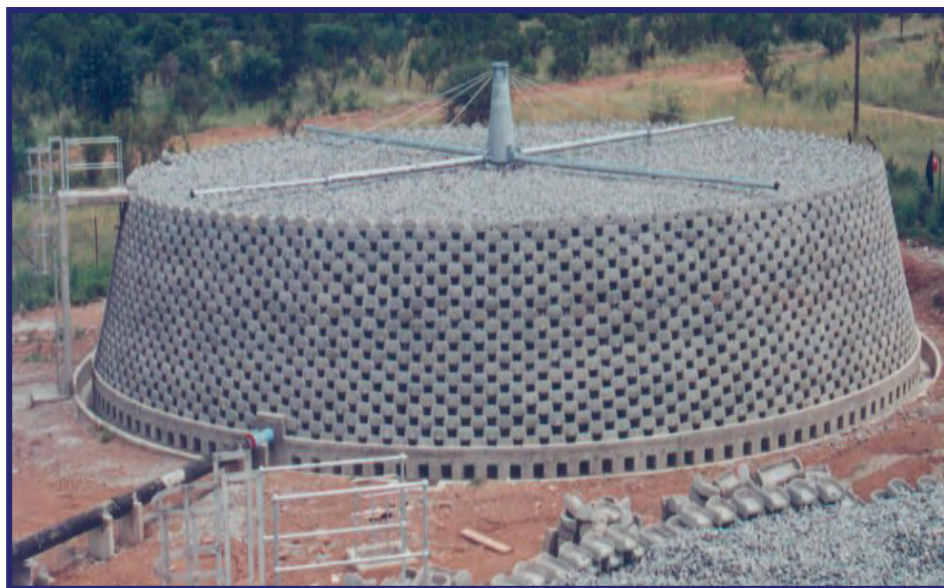
Figure 8.2 (b): Filter Wall Construction Using Interlocking Blocks
