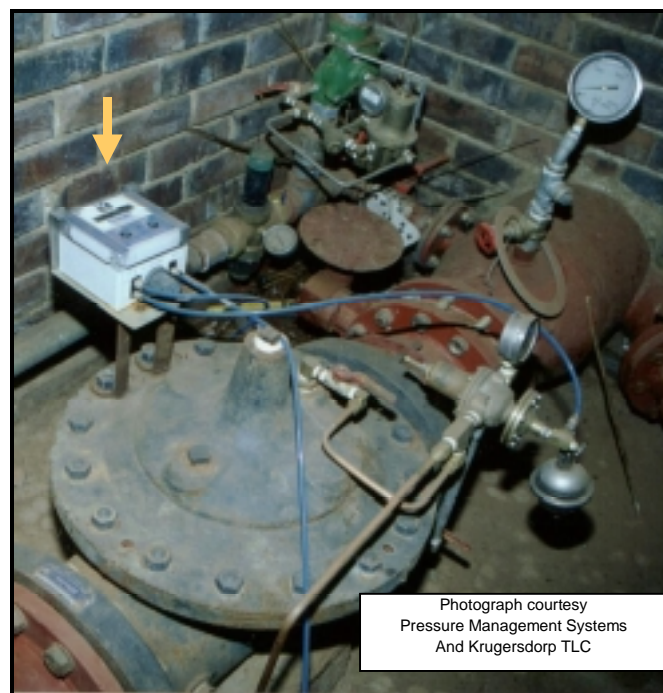
Figure 1.5 : Typical installation of a time-modulated PRV controller
