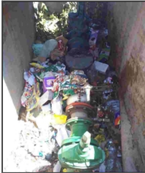
Figure 2.1 : Valve chamber requiring cleaning and securing
