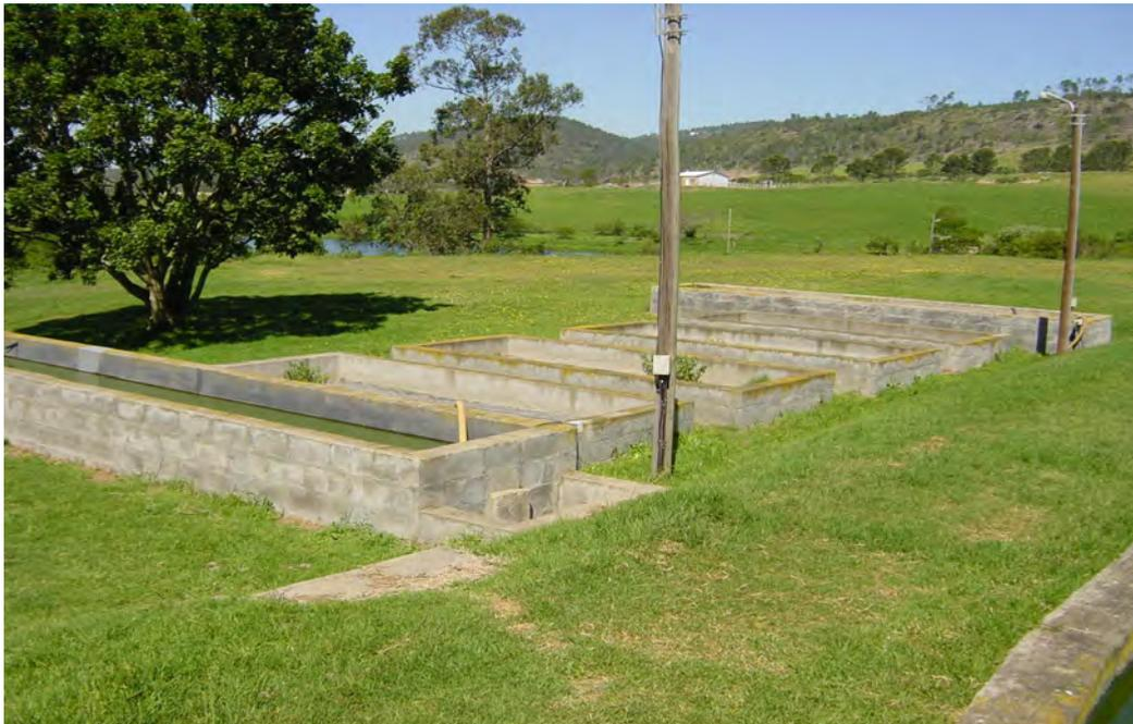
**Figure 3.5:** The four algal drying beds located between the two algal settling ponds.
