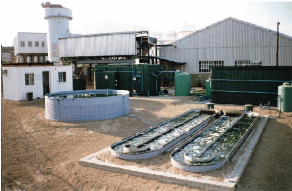
**Figure A7:** Pilot plant at Brennokem Co., in Worcester, South Africa, evaluating the IAPS in the treatment of wine lees and distillery wastewaters.
