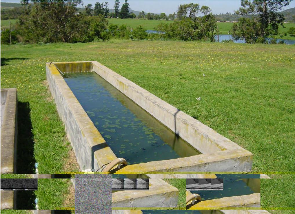
**Figure 3.4:** Algal settling pond with 0.5 day hydraulic retention produces an algal slurry of around 3% solids.
