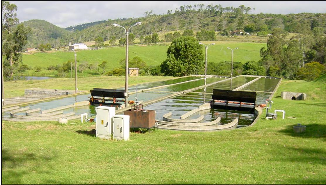
**Figure 3.3:** The high rate algal ponds showing channel dividers used to prevent quiescent zones of flow on the leeward side of the inner pond dividing wall.
