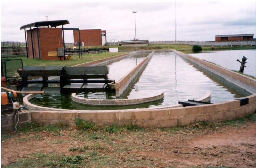
**Figure A6:** The HRAP unit operation of the IAPS plant constructed at the Cato Ridge Abattoir
