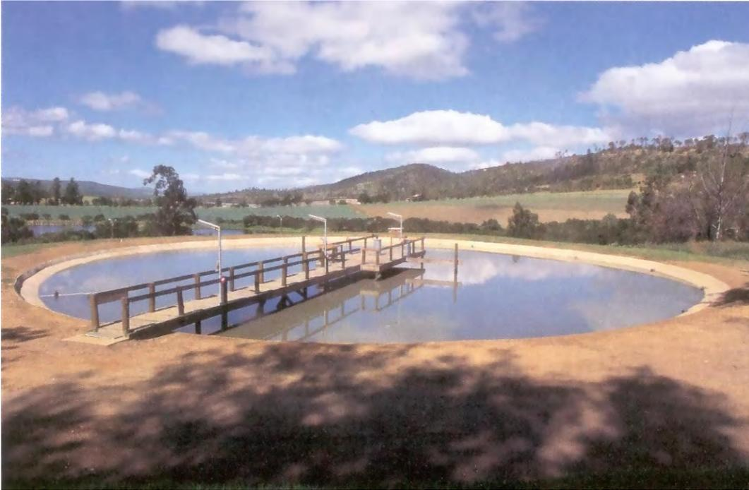
**Figure 3.2:** The primary facultative pond showing the access bridge constructed for access during monitoring and experimental work.
