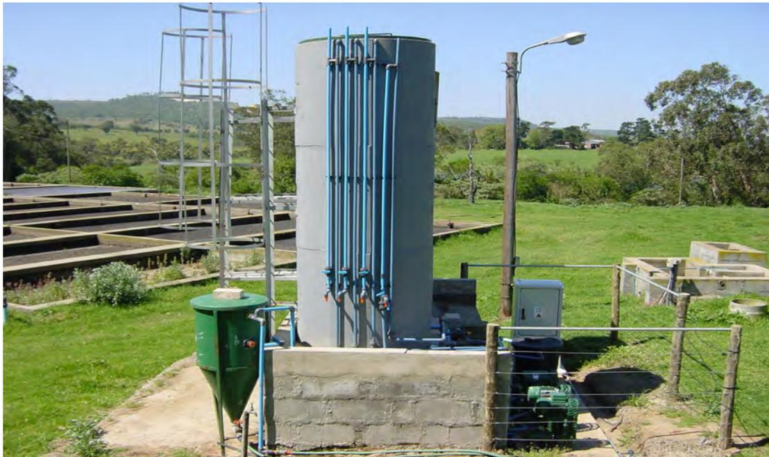
**Figure 9.6:** Stone packed column reactor used for the scale-up evaluation of denitrification studies.
