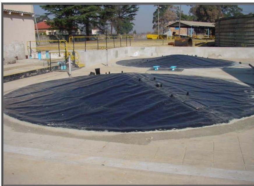
Figure A3.5 The 2 ML scaled-up Recycling Sludge Bed Reactor in the BioSURE ® sewage sludge solubilisation technical-scale plant constructed at ERWAT's Ancor Works in Springs. Surface struts provide supports for a covering membrane.
