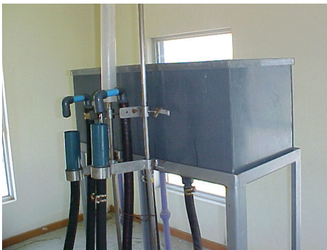
Fig.5 Coagulant dosing systems
