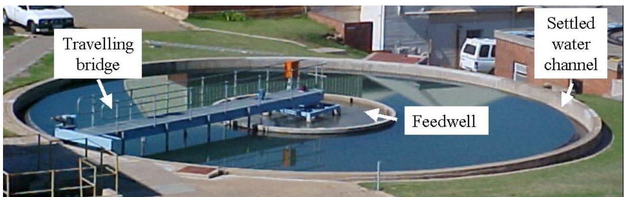
(c) Radial flow clarifier with travelling bridge.
