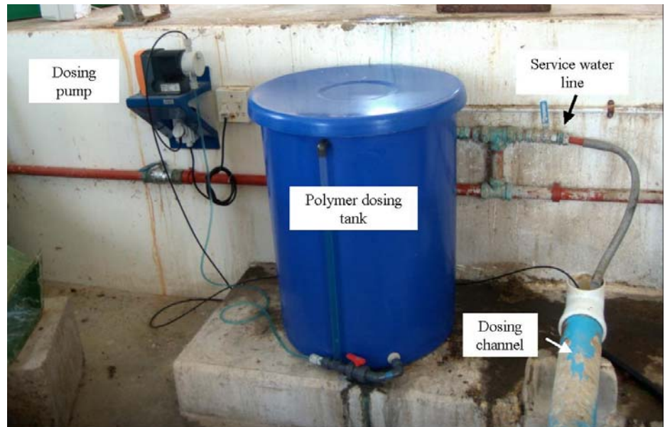
(b) Polymer dosing system with dosing pump.
