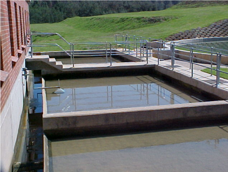
(a) Conventional rapid filters.
