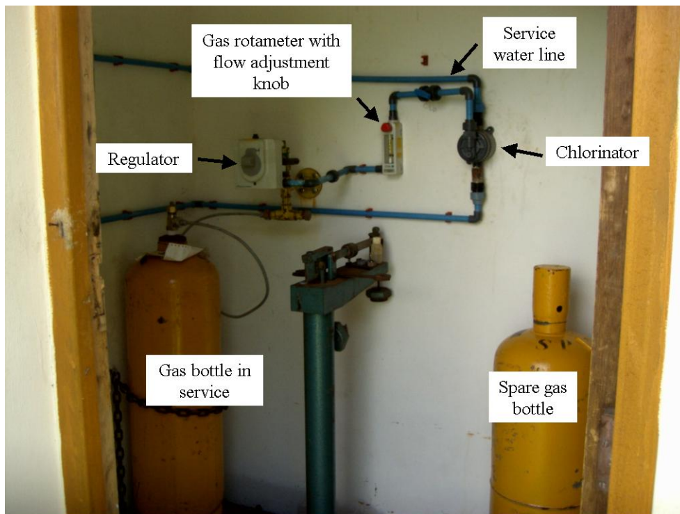
Fig. 2 Gas chlorination system at a small water treatment plant
