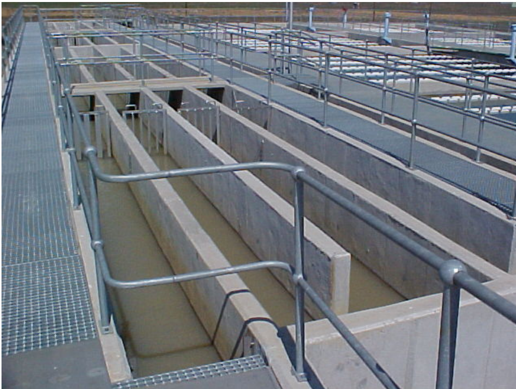
Fig.8 Flocculation channel.
