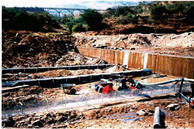
1. SUBSOIL DRAINS UNDER CONSTRUCTION - MASS CONCRETE BASE WITH INVERTED STAINLESS STEEL U-BRACKETS BOLTED TO CONCRETE. 6 mm STONE CONTAINED BY 4.75 X 1.6 mm GALVANISED MESH. 3 X 200 \phi SLOTTED uPVC PIPES CONVEYS WATER TO MAIN PIPE AT BOTTOM OF WEIR (MAIN PIPE NOT SHOWN ON PHOTO).
