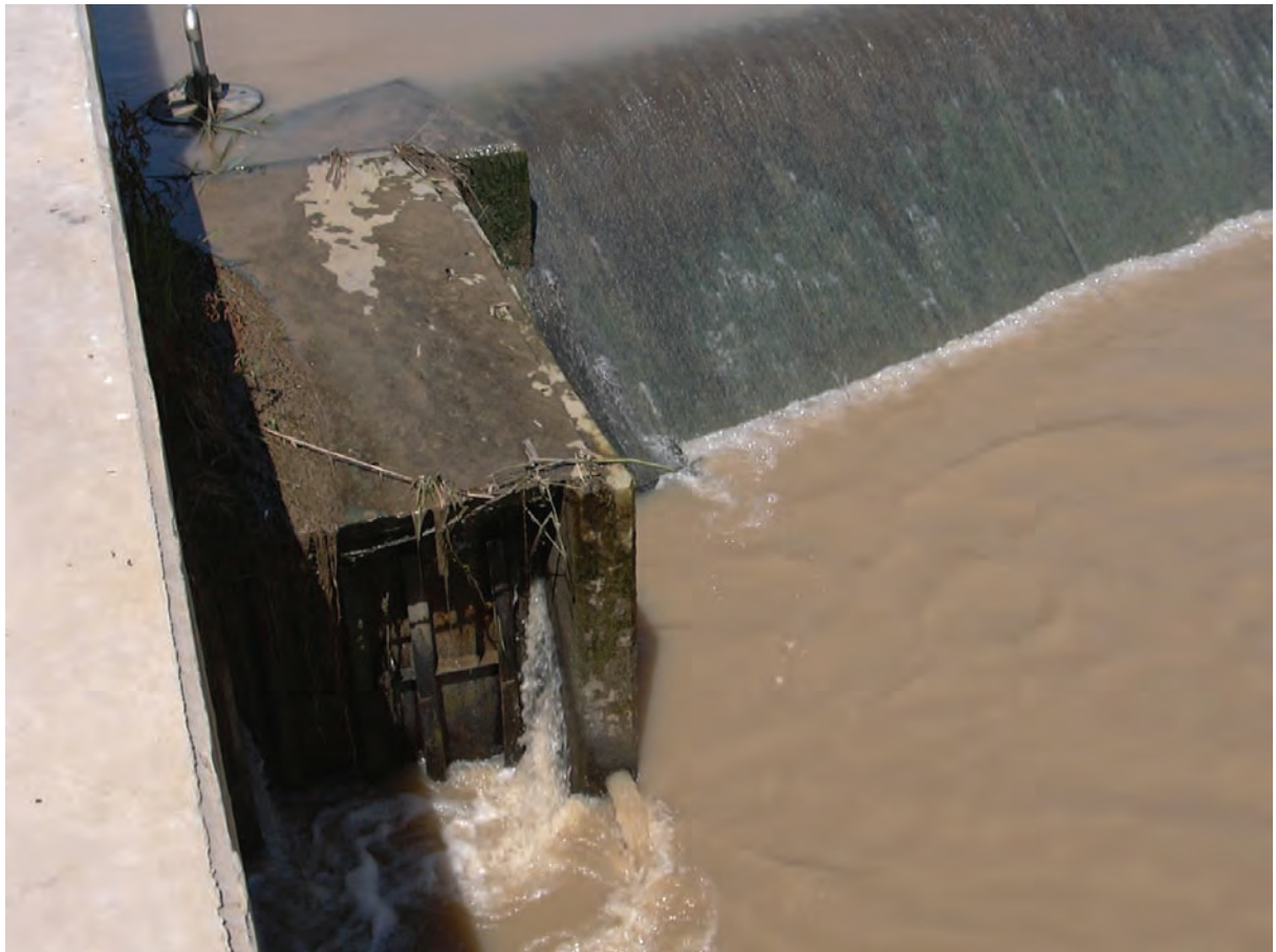
Figure 6-20 Automatic gate viewed from downstream
