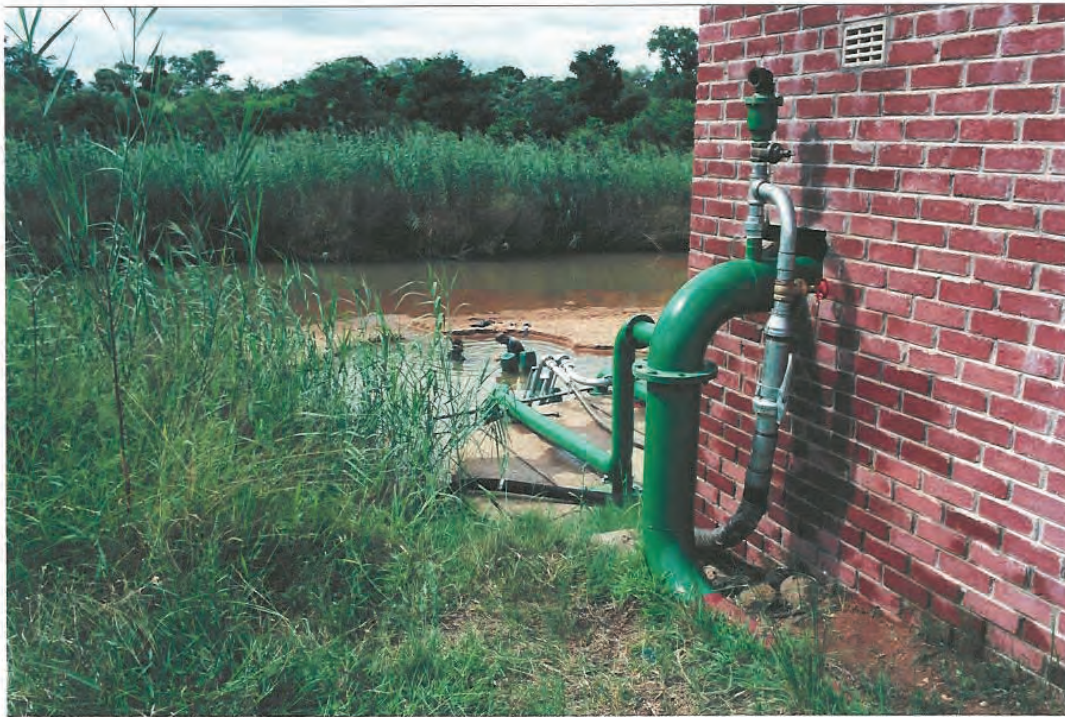
(a) Jet pump motive supply tap off from raw water discharge pipe in foreground and installed fixed jetpump in background.
