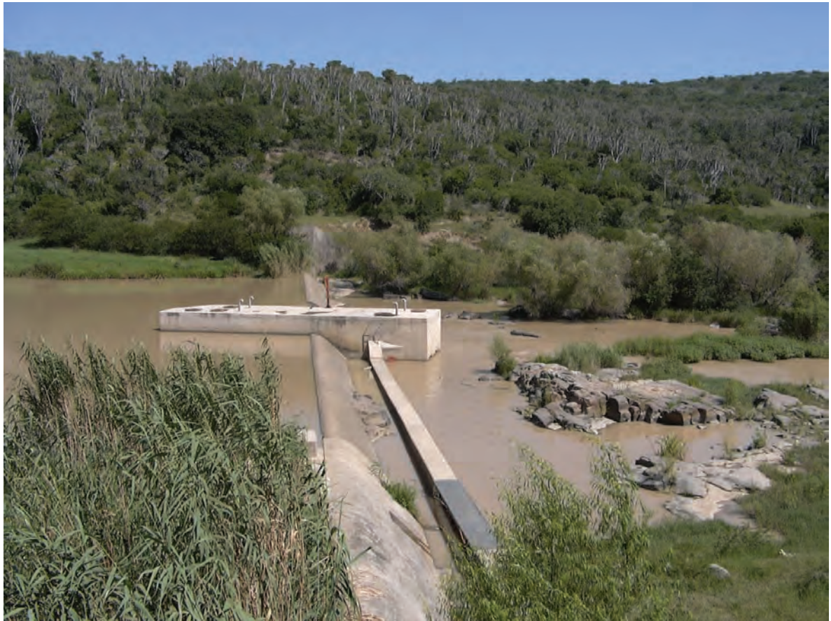
Figure 6-17 Craighead intake structure and weir
