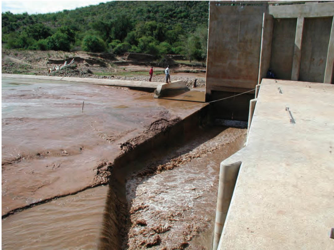
Figure 6-11 Flushing of gravel trap looking downstream
