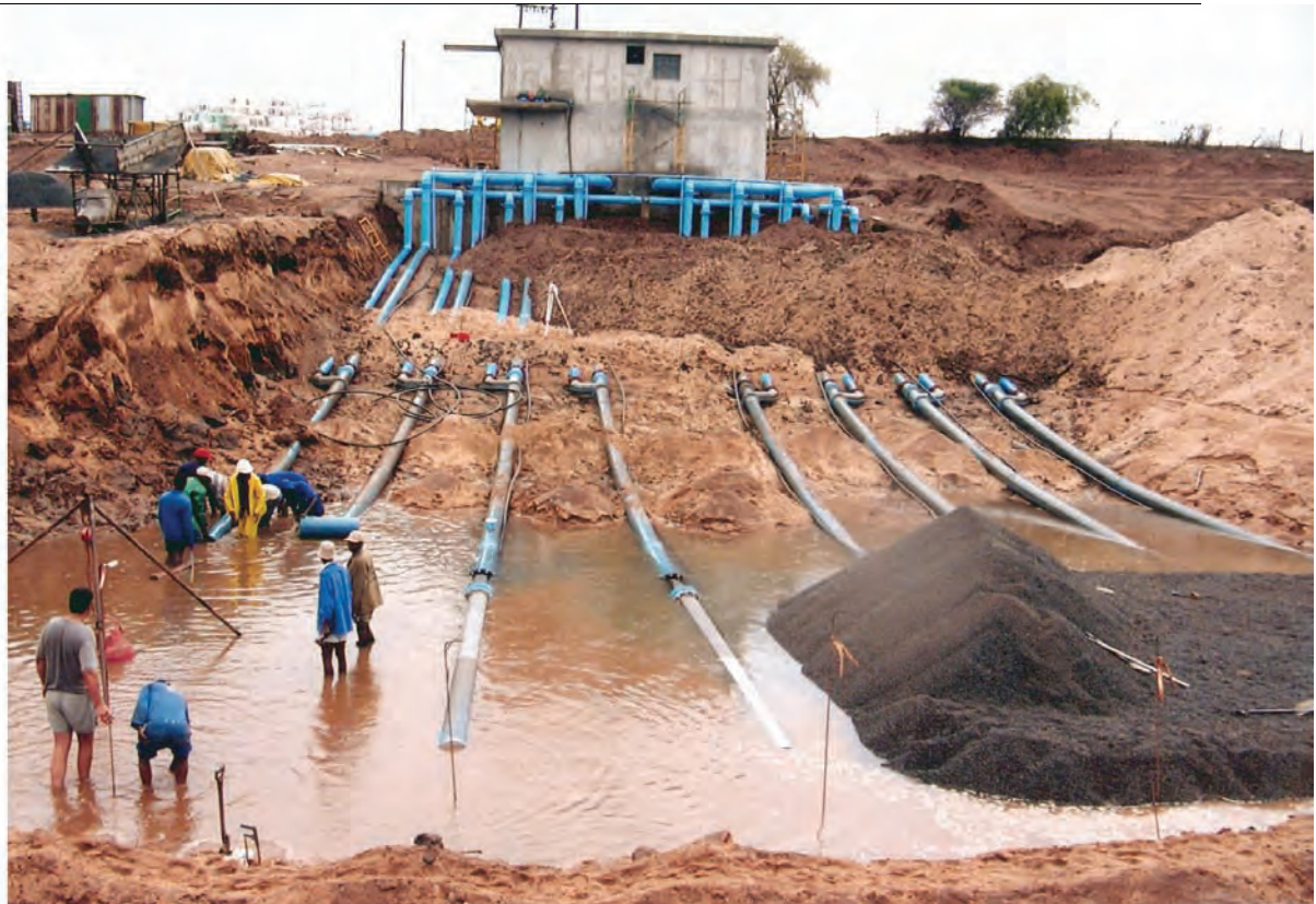
Figure 4 Magudu suction pipe system under construction (Burger du Plessis)
