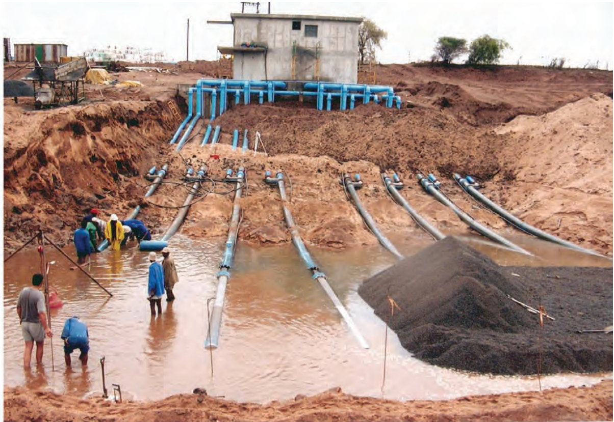
Figure 6-23 Magudu suction pipe system under construction (Burger du Plessis)
