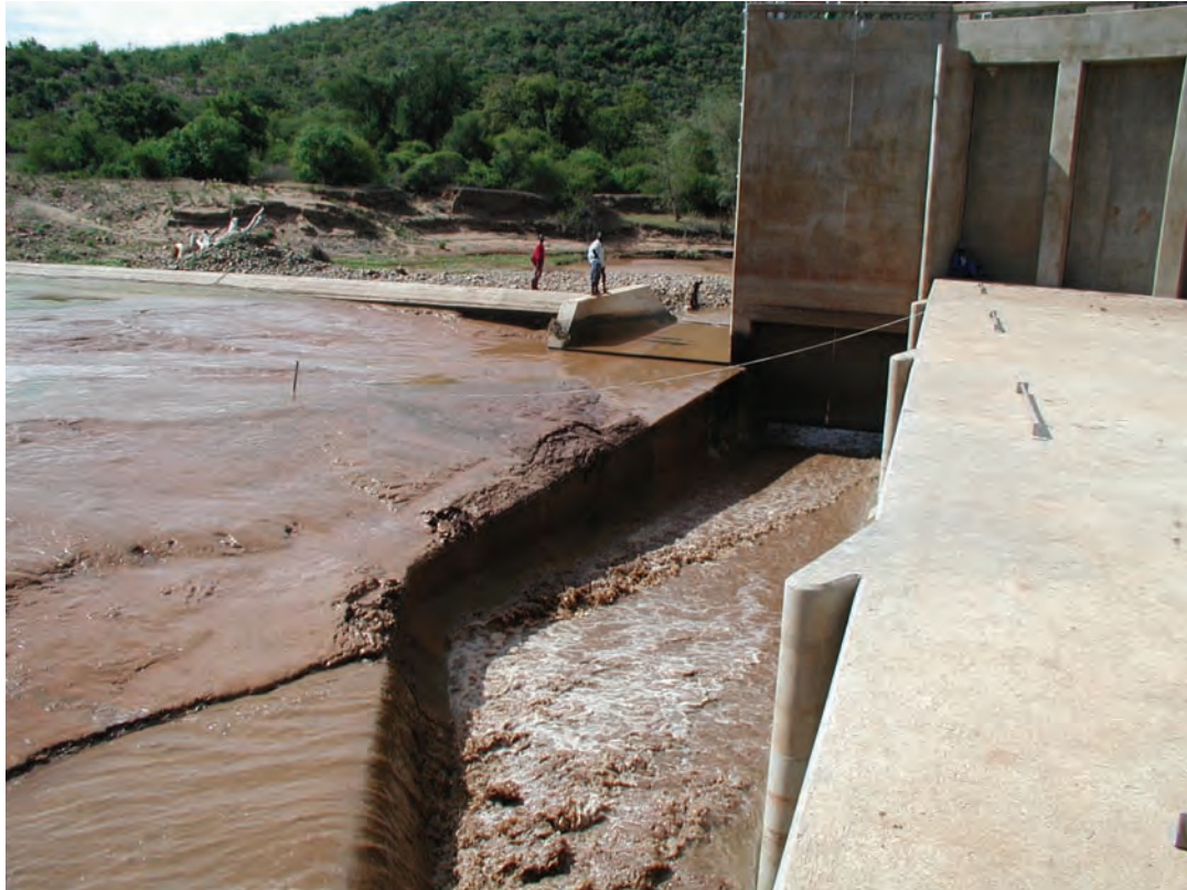
Figure 3 Flushing of gravel trap looking downstream
