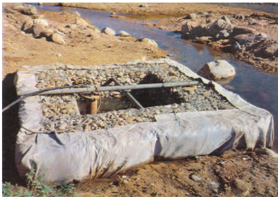
Figure 6-21 Small pumpstation consisting of gabion boxes and concrete slab
