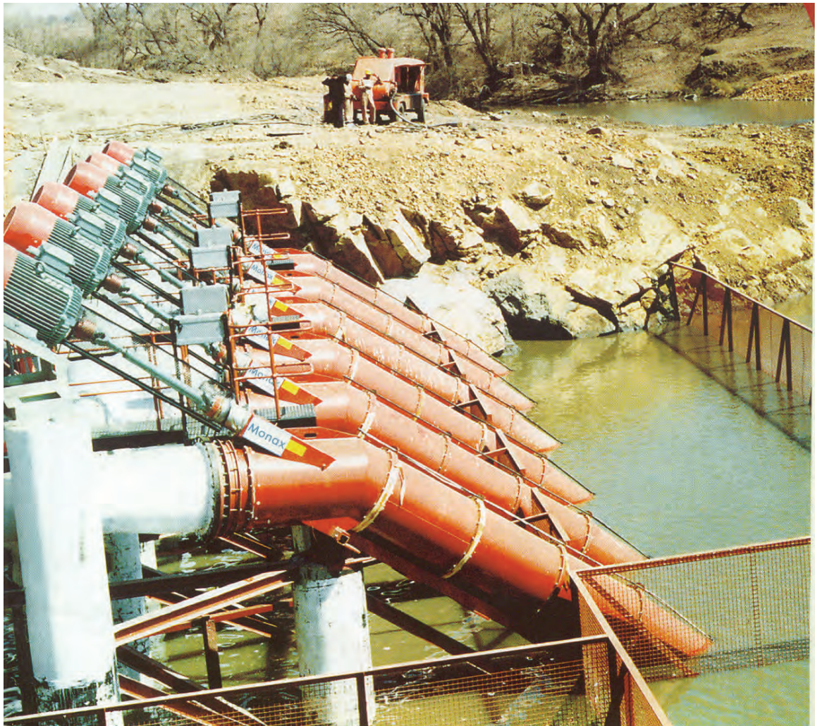
Figure 6-2 Axial flow low lift pumps
