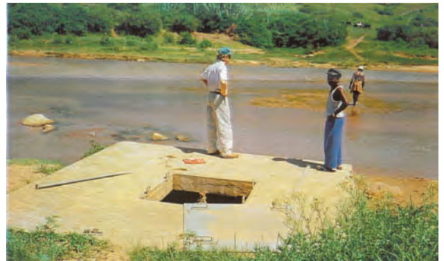
Figure 6-21 Small pumpstation consisting of gabion boxes and concrete slab
