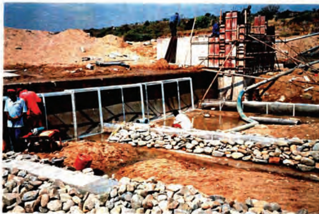
2. 3 x SUBSOIL DRAINS BEING COVERED WITH BOULDERS FOR FURTHER PROTECTION AND IMPROVED FILTRATION. PRIMARY COLLECTION CHAMBER UNDER CONSTRUCTION.
