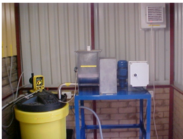
Figure 5.7: Powder Feeder and Fluoride Saturator System
