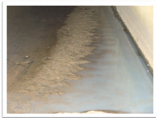
Figure 5-11 Liesbeek River: Milky discharge in stormwater outlet
