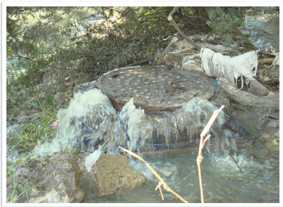
Figure 3-3 One of nine overflowing sewerage manholes prior to the Cycle Park (Source: Author)
