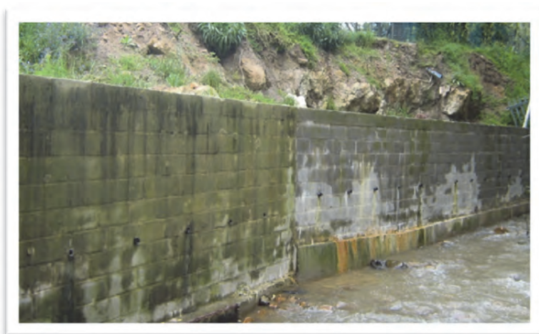
Figure 3-24 Engineered bank armouring covering 100% of the bank
