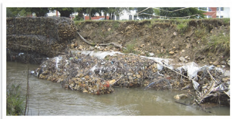
Figure 3-23 Example of cut bank where gabion has failed
