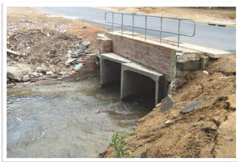
Figure 3-43 Inadequate capacity culvert bridge damaged by excessive flows
