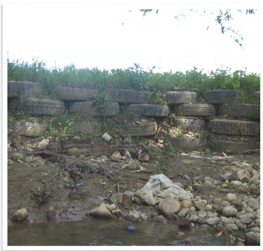
Figure 3-37 Stacked tyres as a levee to prevent flooding of the floodplain, Wellington, Western Cape
