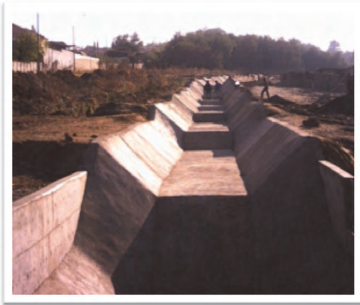
Figure 3-33 Canal constructed to divert a stream around a housing complex, Gauteng
