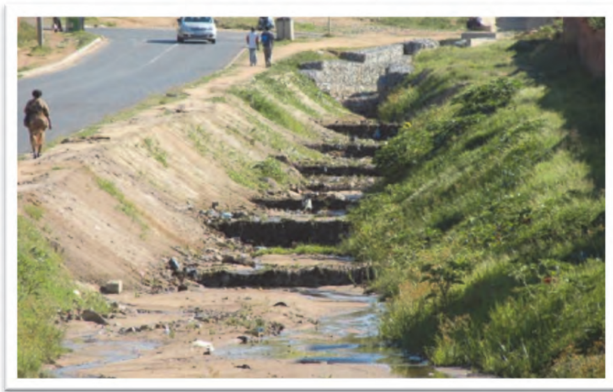
Figure 3-35 Sustainable urban designed (SUD) stormwater canal
