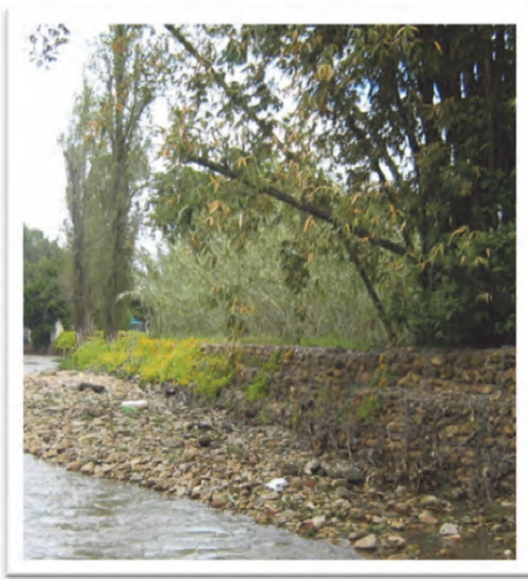
Figure 3-25 Armoured bank with gabion baskets
