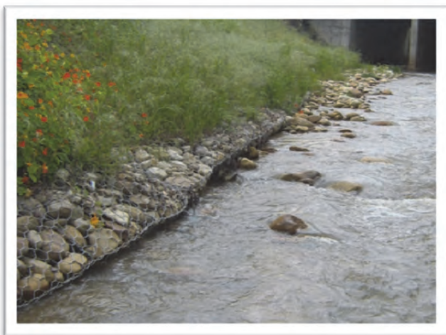
Figure 3-27 Bank toe armouring using gabion baskets
