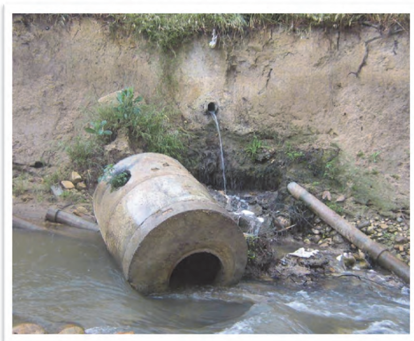
Figure 3-30 A sewer in a poor state
