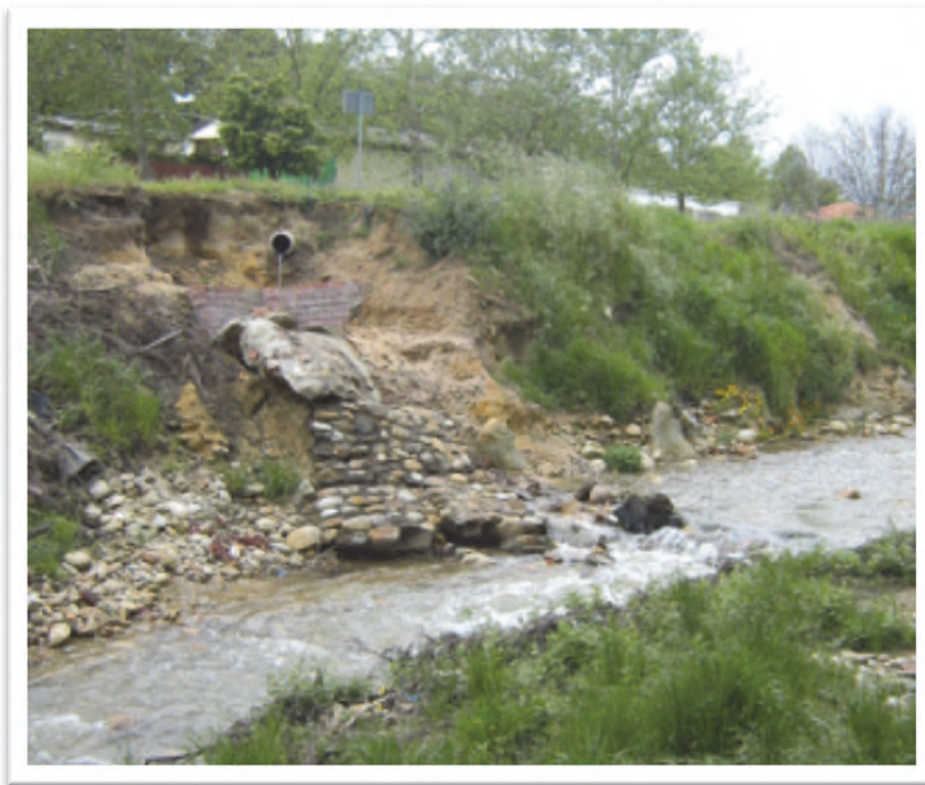
Figure 3-29 Collapsed stormwater outlet
