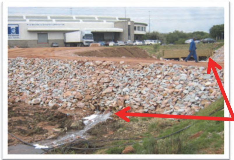
Figure 3-41 In-stream impoundment, where the inflow exceeds the outflow capacity
