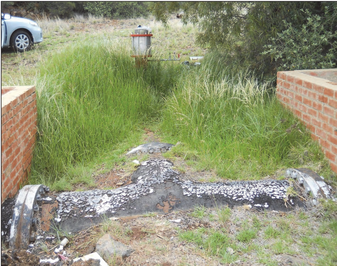
Figure 4-31: Set-up point at upstream of T-piece at air valve
