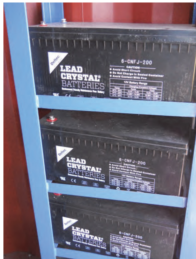
Figure 5-35: Battery bank
