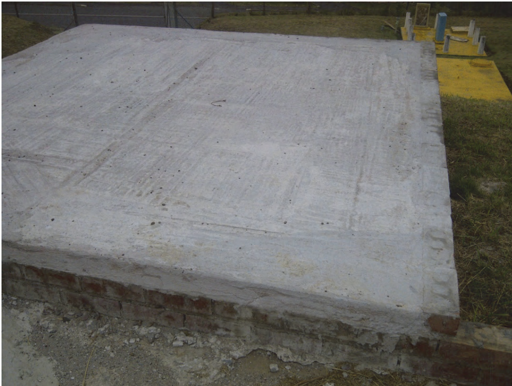
Figure 5-16: Concrete floor for hydropower plant
