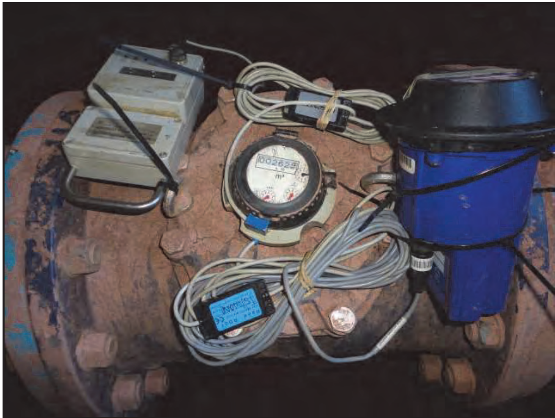
Figure 3-26: GSM wireless logger connected to flow meter
