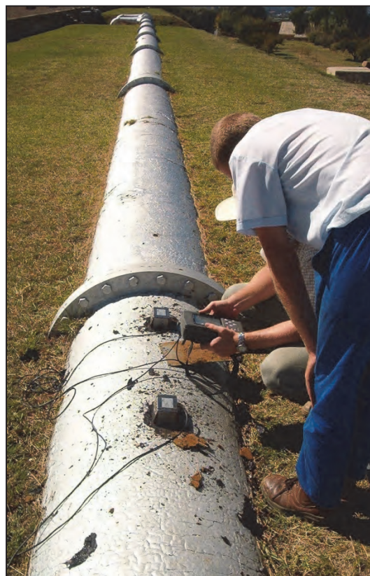
Figure 4-18: Flow meter installation
