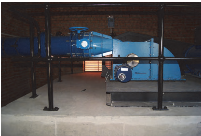
Figure 4-56: Completed turbine installation
