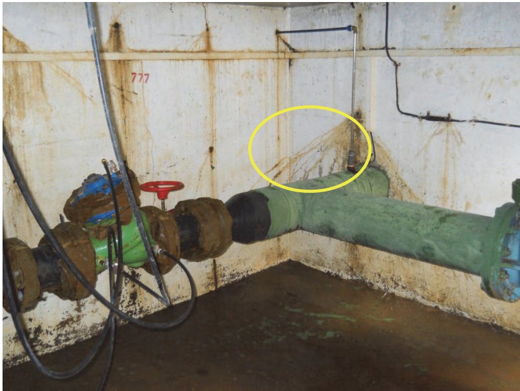
Figure 5-13: Initially proposed location of off-take within PRS chamber
