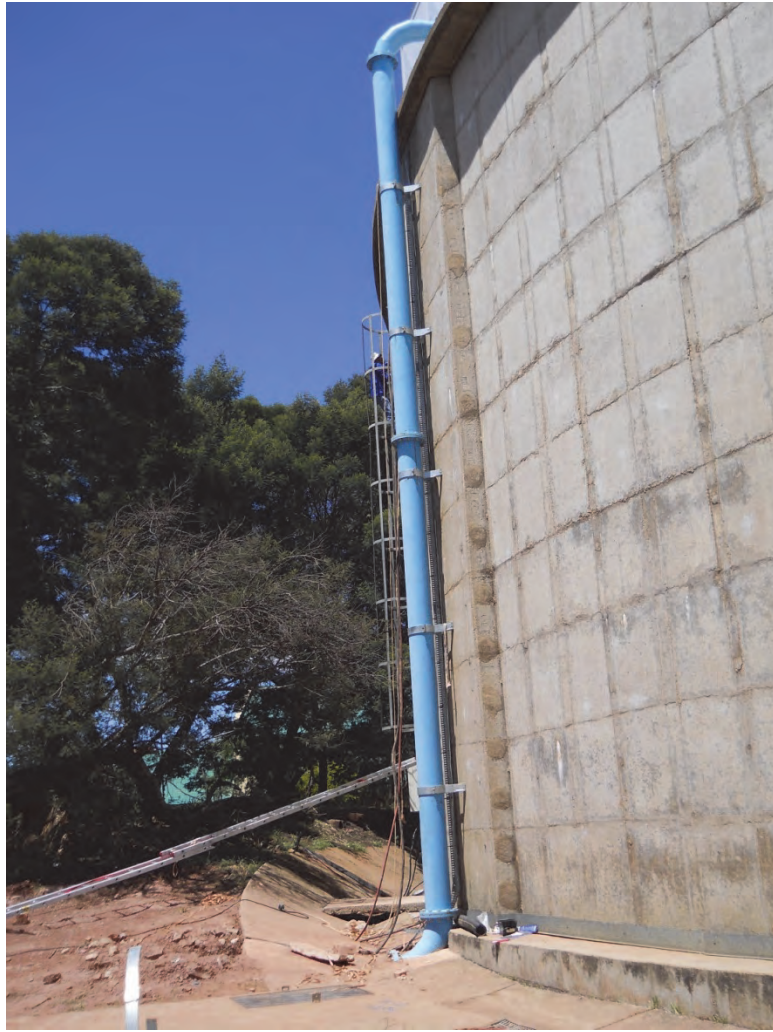
Figure 3-59: Completed turbine supply line on to top of reservoir
