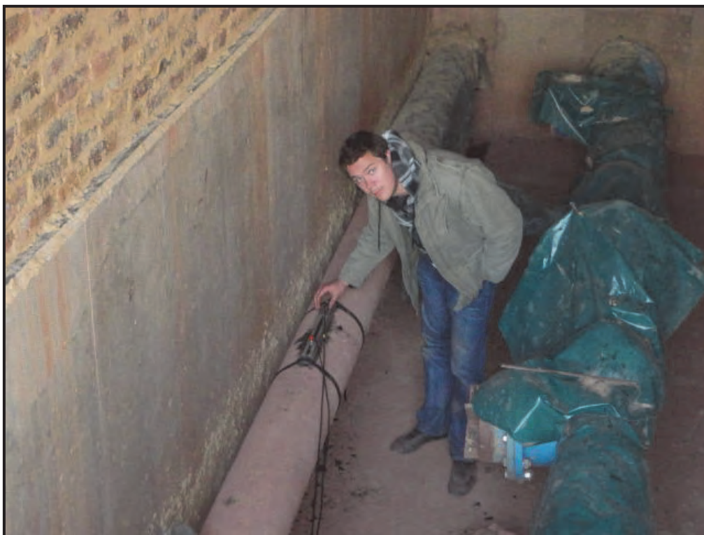
Figure 3-11: Set-up of flow meter
