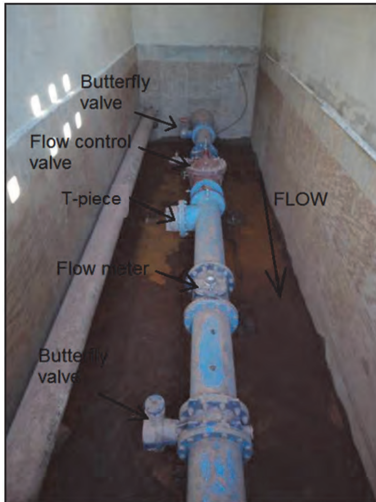
Figure 3-23: New valve chamber set-up
