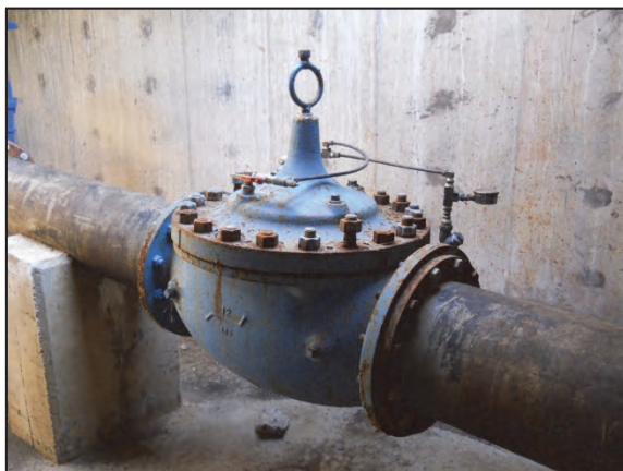
Figure 6-27: Control valve at Sandile WTW
