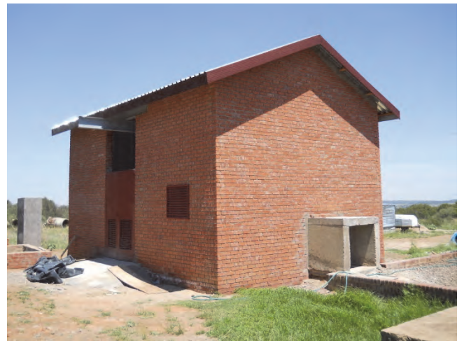
Figure 4-47: Turbine room almost complete
