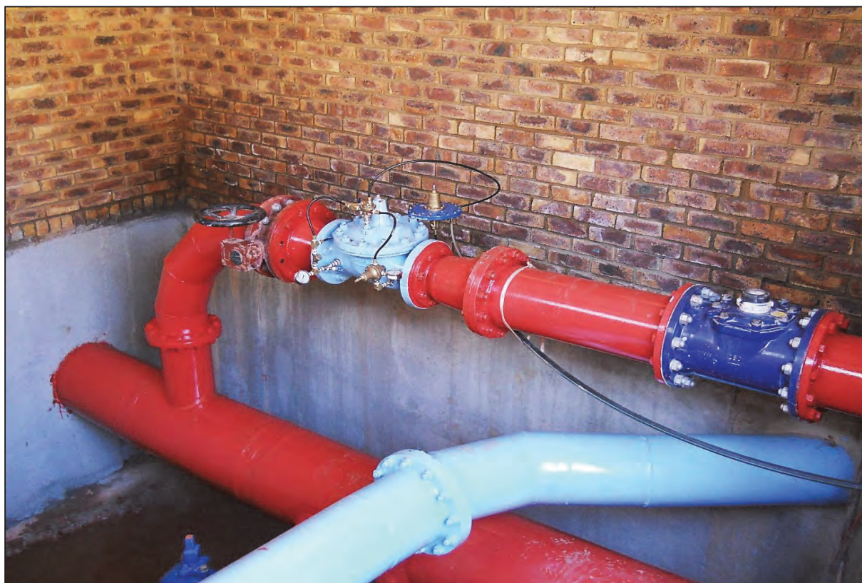
Figure 3-47: Completed off-take pipework
