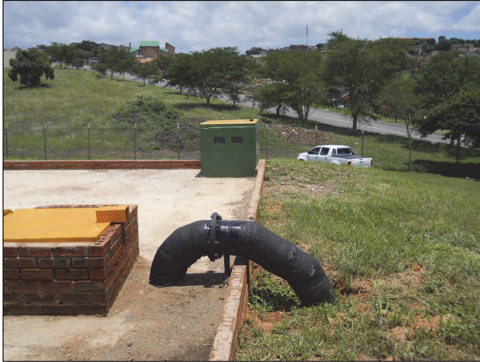
Figure 5-12: Discharge point into the top of the reservoir (photograph taken before constructed hydropower station)
