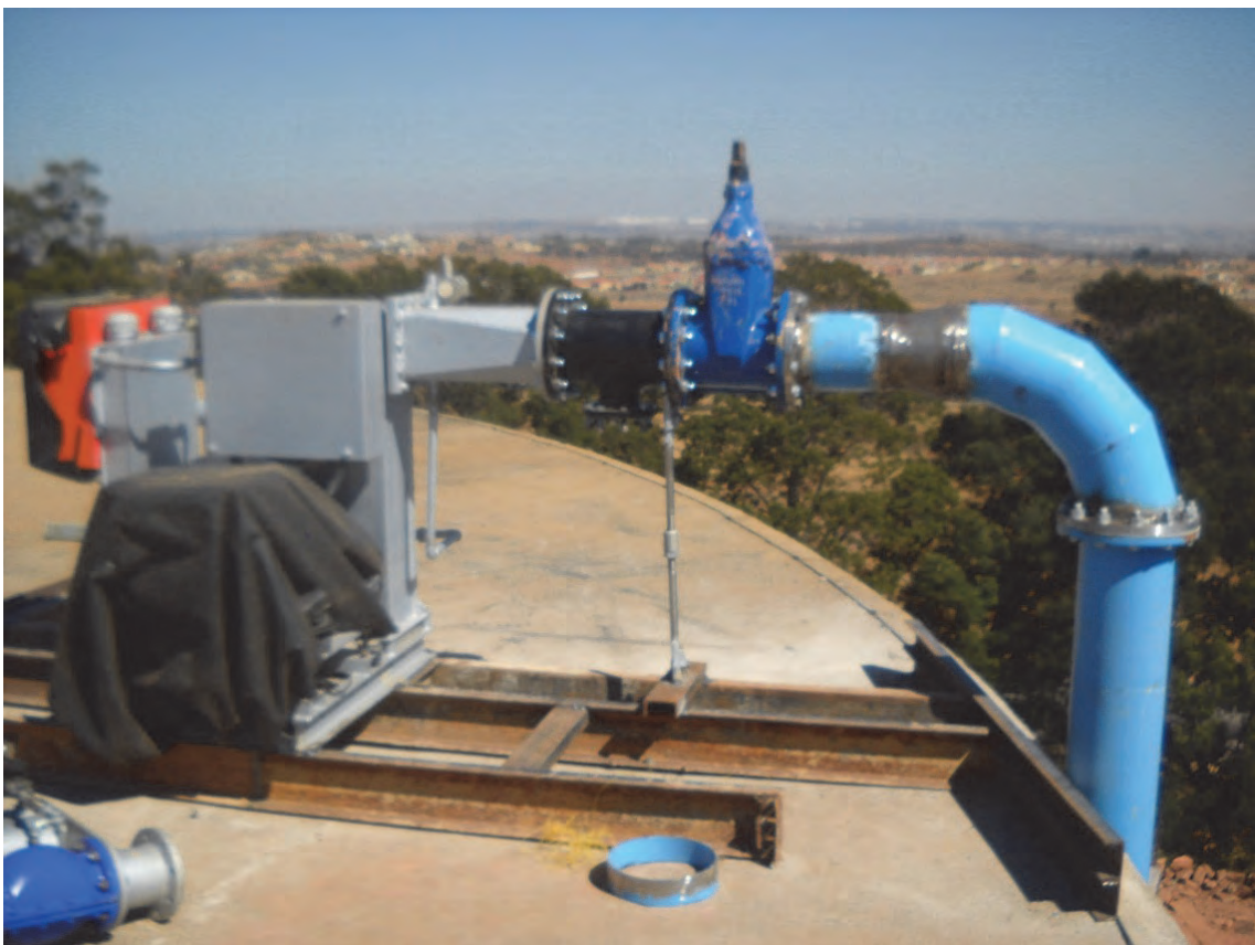
Figure 3-63: Crossflow turbine installation (connecting to supply line)
