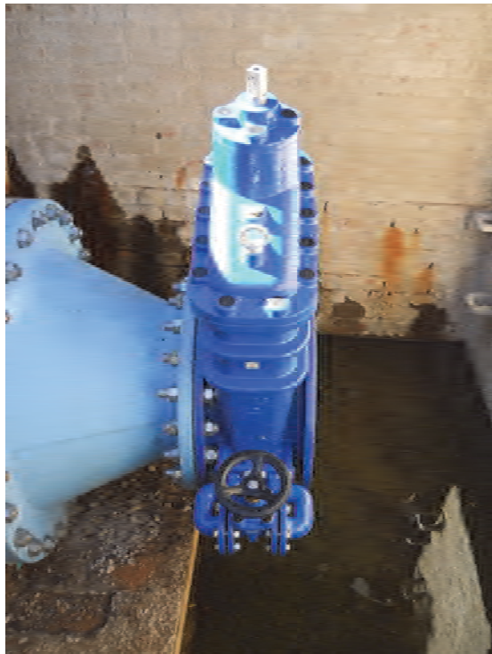
Figure 4-48: Connection point fitted with reducer and isolating valve
