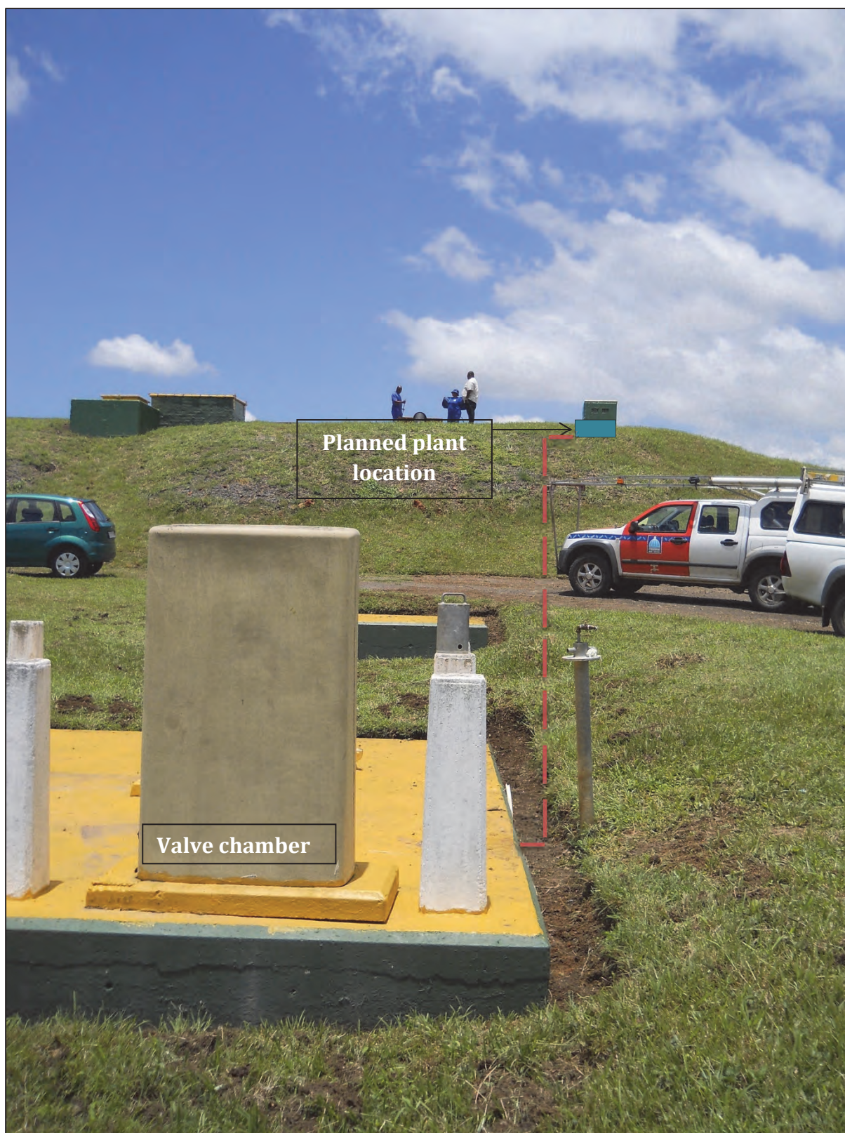
Figure 5-9: Pipe excavation (red) and location for pilot plant
