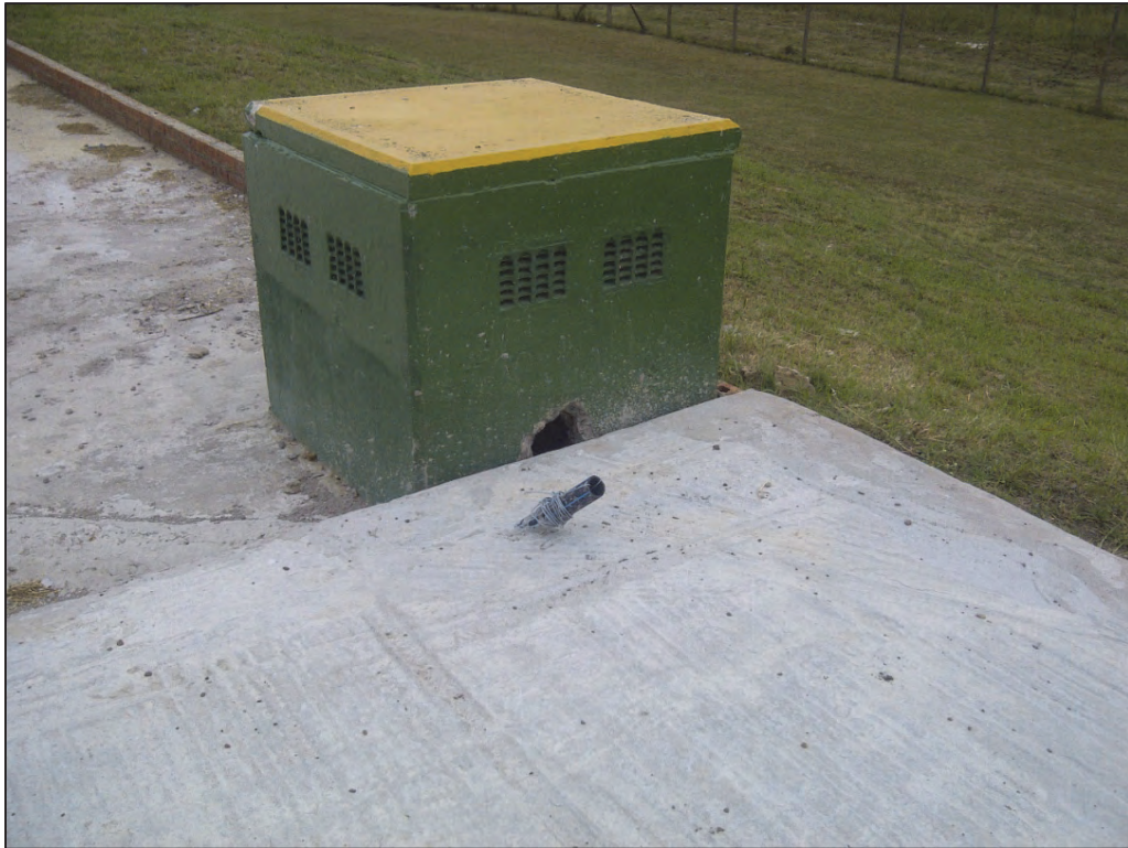
Figure 5-17: Connection into air vent
