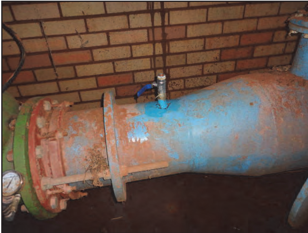
Figure 3-8: Pressure tapping welded onto bulk pipe
