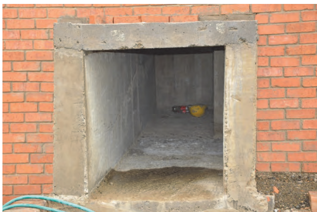
Figure 4-60: Outlet canal into reservoir
