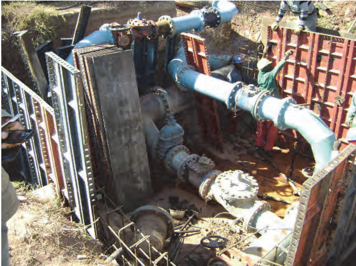
Figure 3-57: Constructing the off-take chamber
