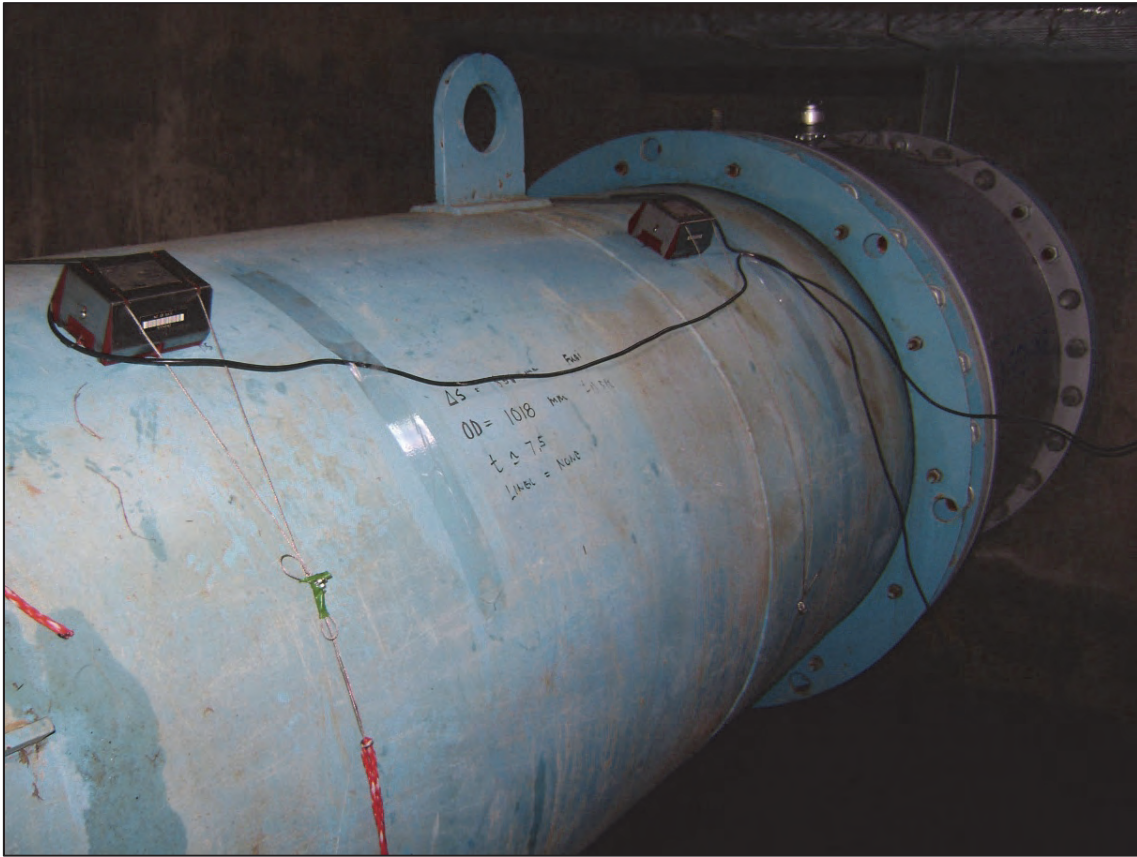
Figure 4-14: Ultrasonic flow meter installation
