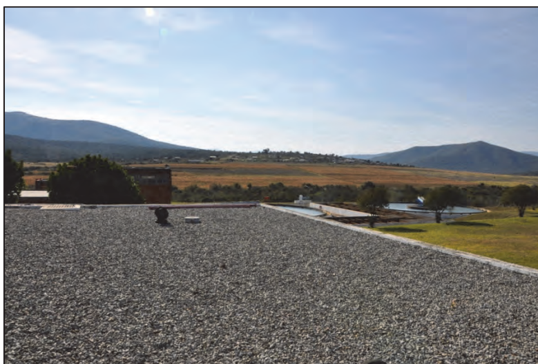
Figure 6-28: Balancing tank at Sandile WTW
