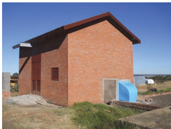
Figure 4-61: Turbine room with chute into top of reservoir
