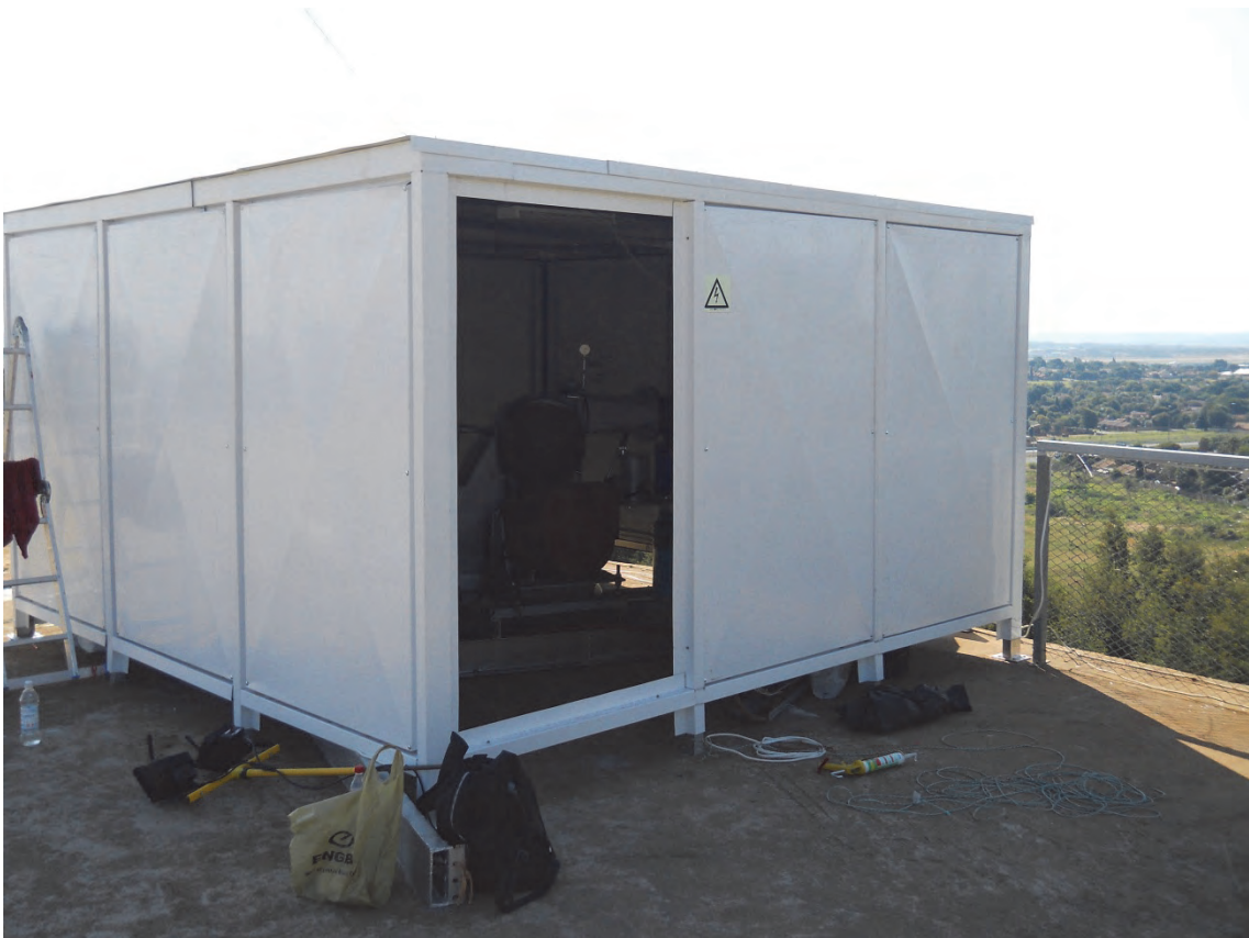
Figure 3-69: Pilot plant enclosure
