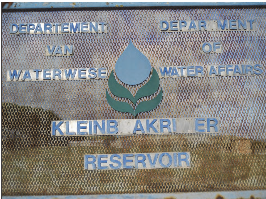
Figure 6-13: Klein Brak Reservoir which supplies Klein Brak WTW
