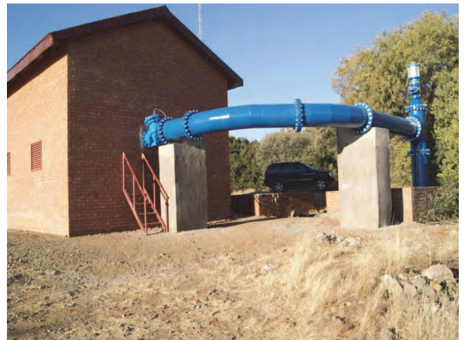
Figure 4-51: Off-take linking into turbine room
