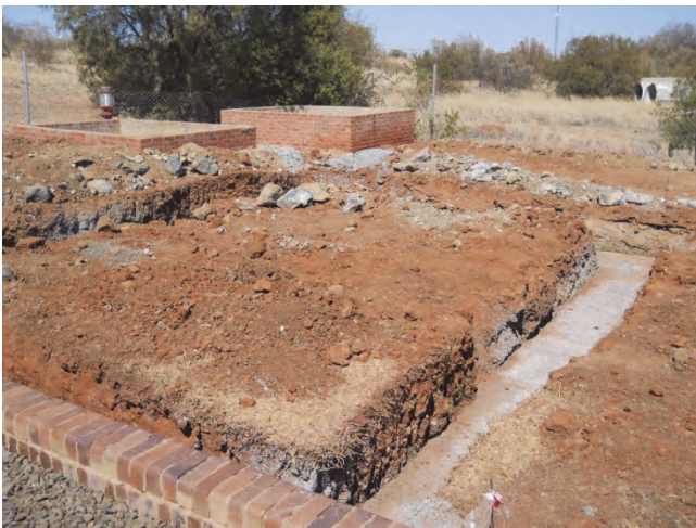
Figure 4-46: Turbine room foundation
