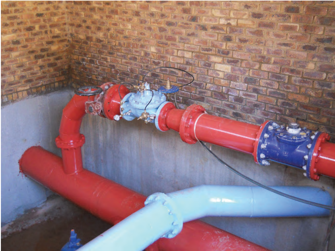
Figure 3-60: Completed off-take chamber pipework
