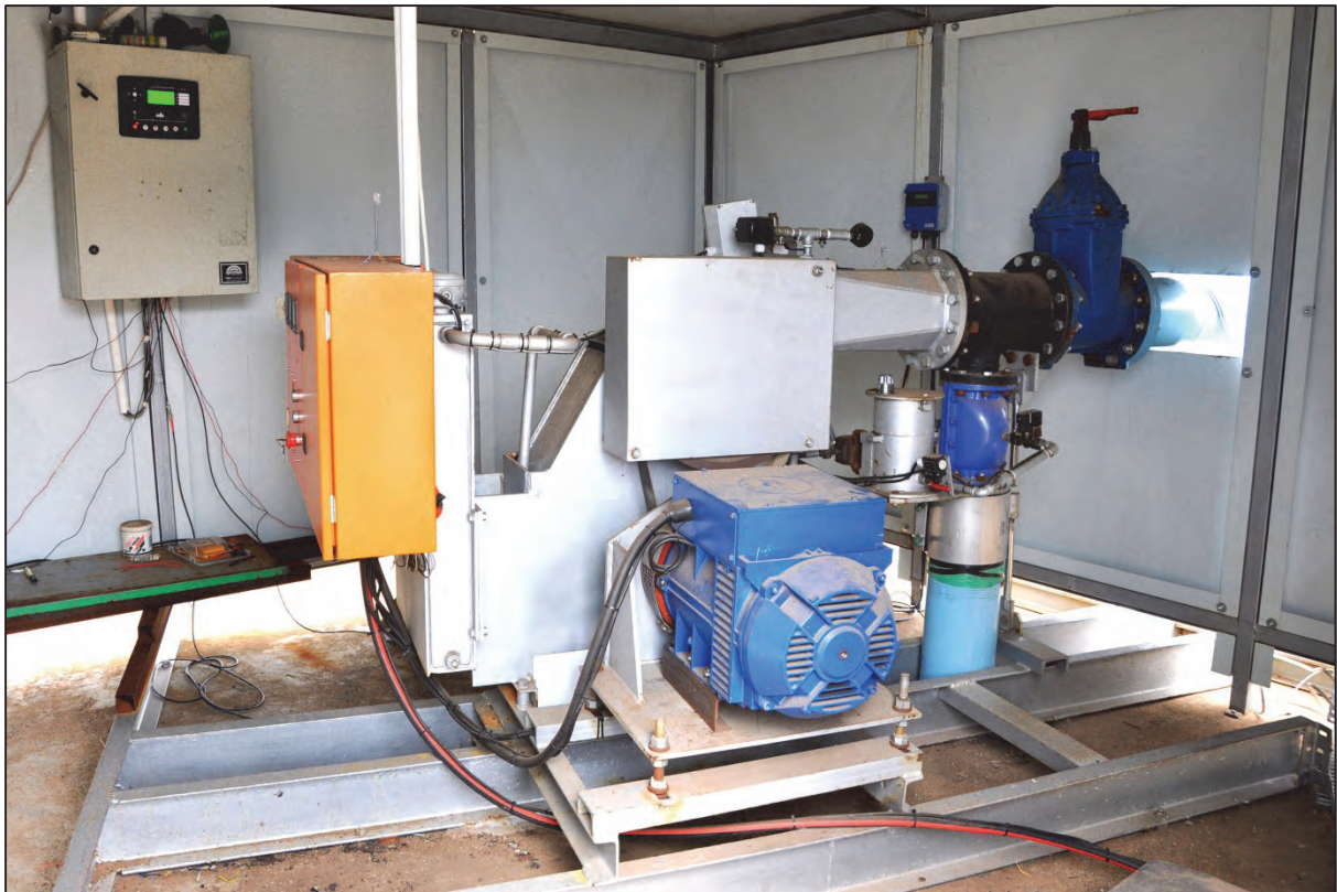
Figure 3-48: Completed turbine on steel-beam supports
