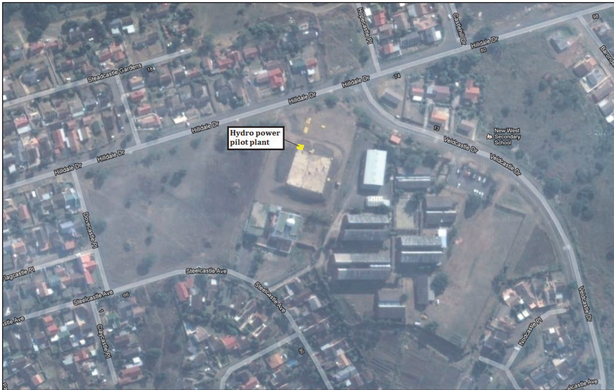
Figure 5-7: Aerial view of Newlands 2 Reservoir site
