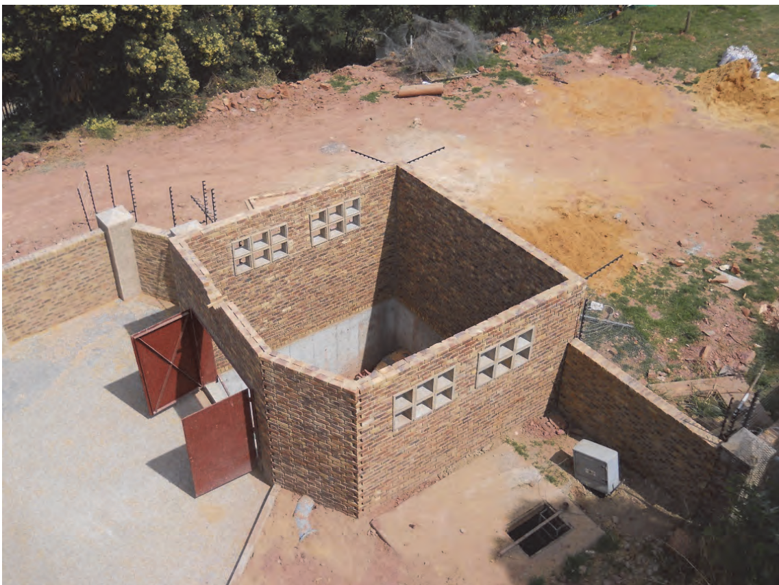
Figure 3-58: Nearly complete off take chamber (Pierre van Ryneveld Reservoir)
