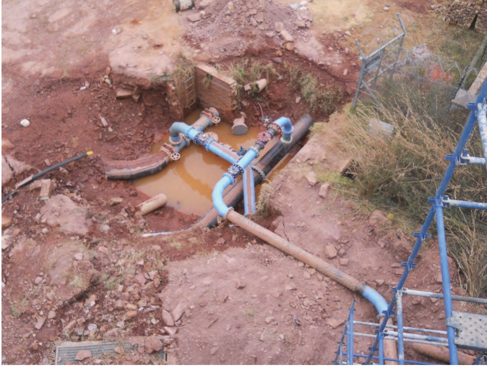
Figure 3-55: Plan view of off take pipework
