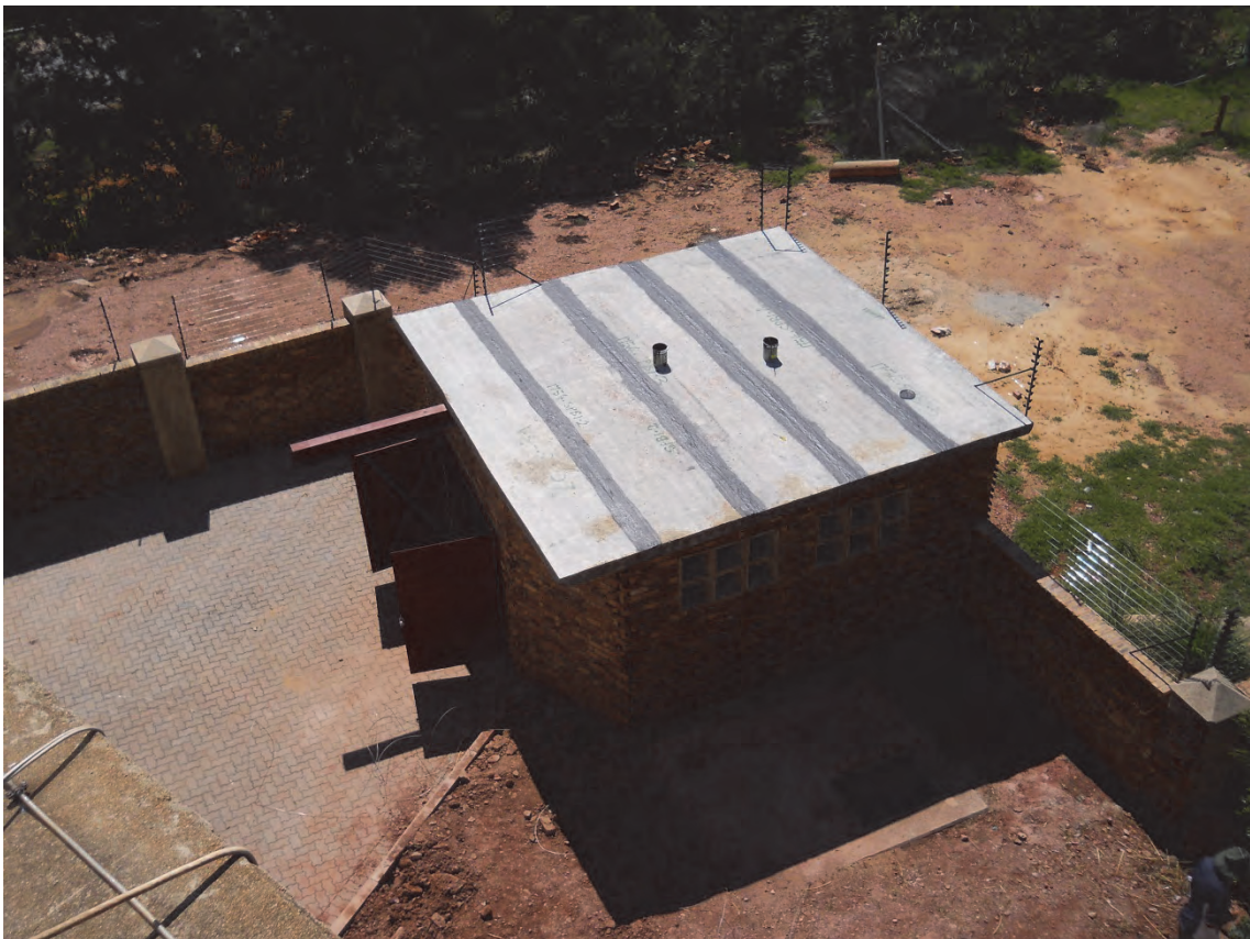
Figure 3-61: Completed off take chamber
