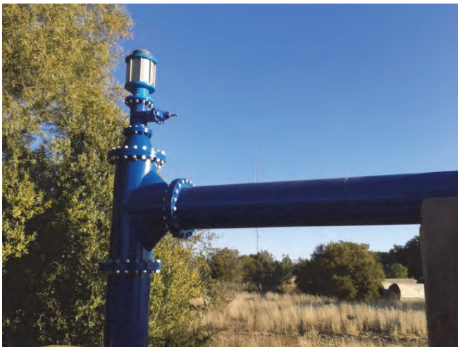
Figure 4-50: Air valve on off-take for effective deaeration
