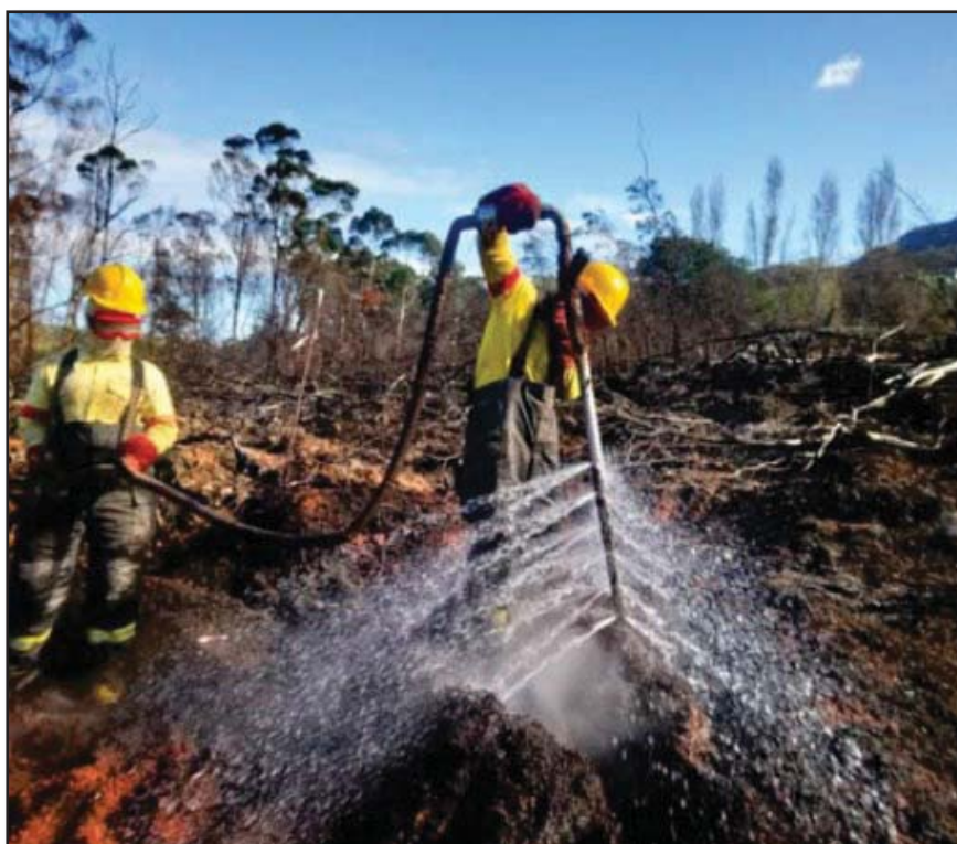
Figure 4.2 The spike tool designed to extinguish peat fires (Grundling et al., 2019).
