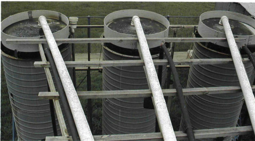
A top view of the Pilot Plant biofilters. The three biofilters were packed with three different media size fractions: small, medium and large.
