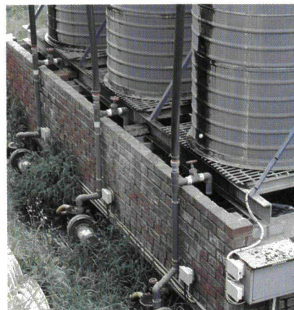
The recirculation pump installations seen at the back of the biofilters.
