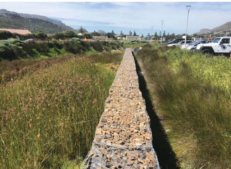
Figure 17. Wet detention pond with forebay at this shopping centre parking area allows stormwater attenuation and water quality purification. (Credit: Liz Day)
