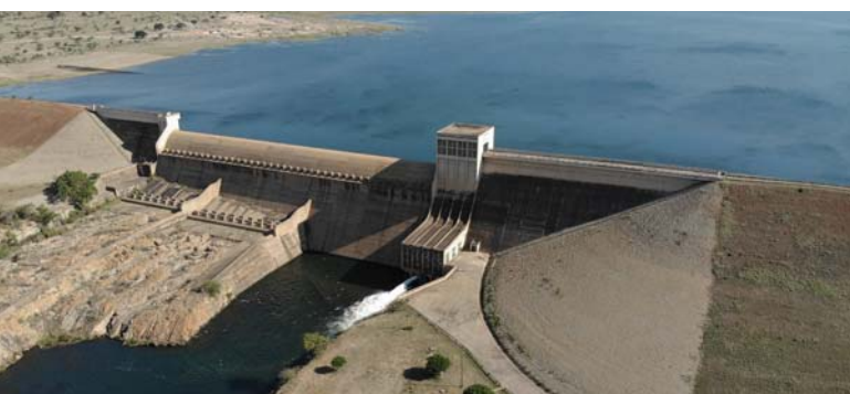
Figure 11. Driekoppies Dam, Lomati River, completed in 1997. (Credit: Rob Palmer)
