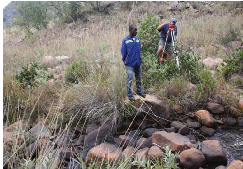
Figure 8. DWS staff conducting a hydraulic survey in the upper Matlabas River for a rapid EWR study in the Marakela National Park Limpopo. (Credit: Christa Thirion)
