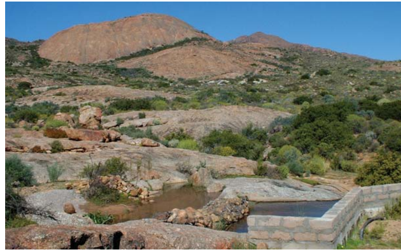
Figure 10. The simple sand filter in the bed of the river, which flows through a valley carved from granite at the Karkams artificial recharge scheme. (Credit: Water Wheel archives)
