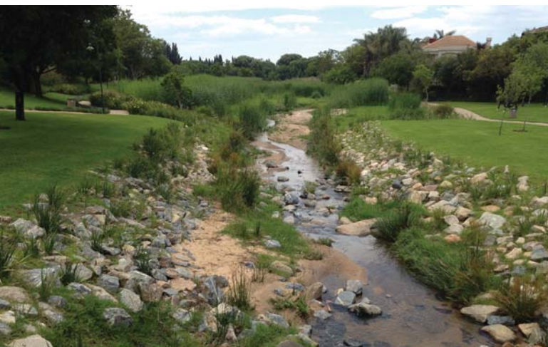
Figure 20. Fourways: Rehabilitation of an incised urban tributary of the Jukskei River, Fourways Gardens, Gauteng. (Credit: Liz Day)
