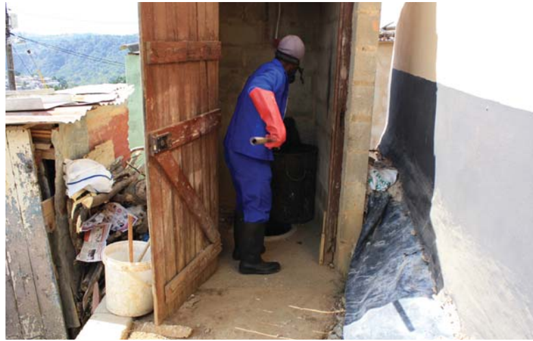
Figure 14. Manual pit emptying taking place in eThekweni Metro. (Credit: Lani van Vuuren)
