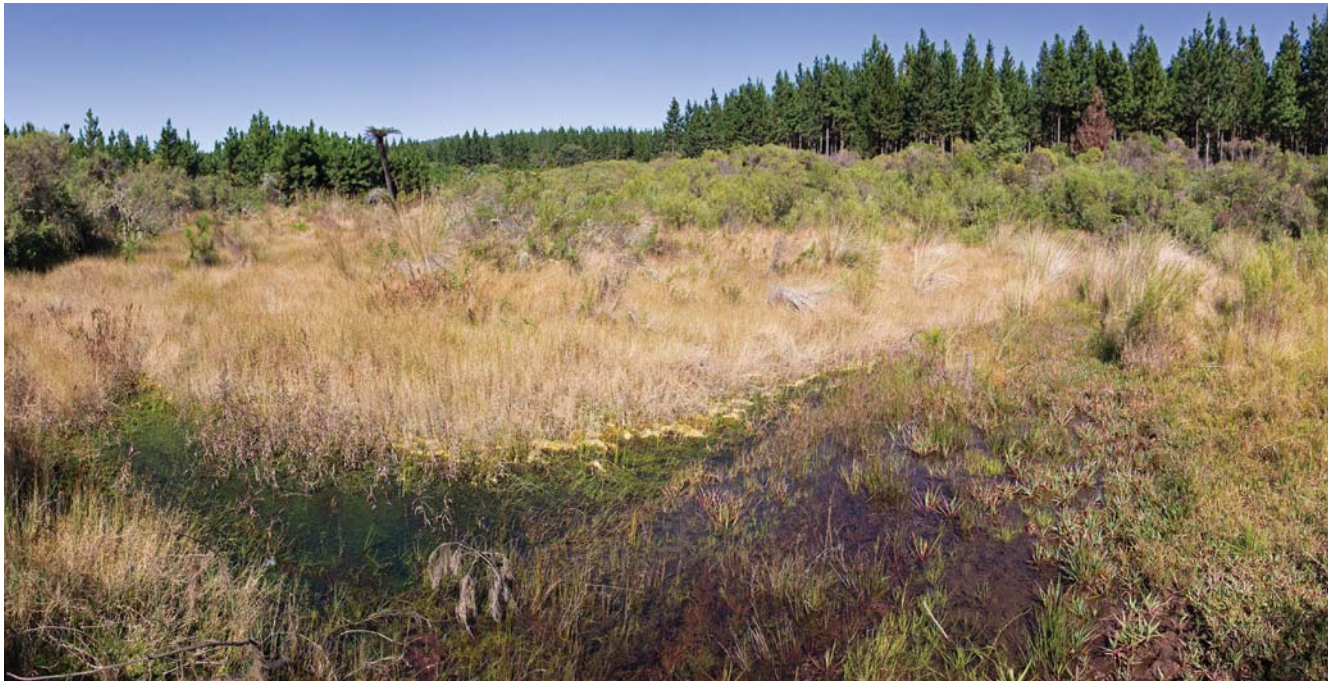
Figure 8: The Mutale Peat Wetland looking upstream from the road culvert. The photograph shows pond formation caused by the culvert, pine trees establishing within the wetland, Passerina montana dominated bush encroachment on the upper banks and pine plantations surrounding it.
