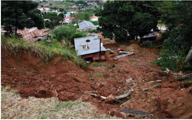
It cost billions of Rand to repair the provincial and national road infrastructure damaged by the floods.
