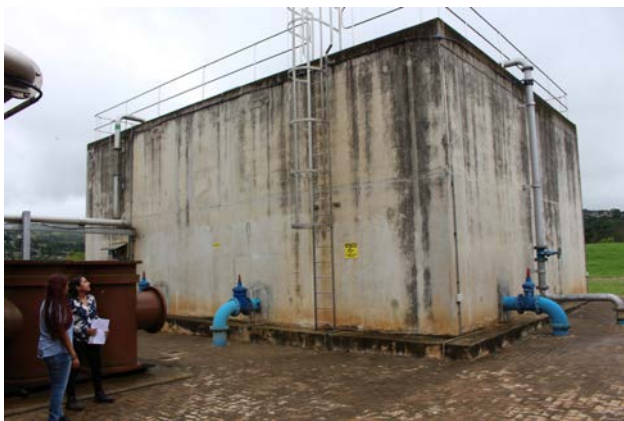
Treated water, the end product of the reuse project, is stored in a 600 000-litre reservoir for supplying process water to Darvill Wastewater Treatment Works.
