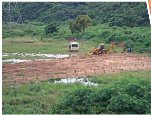
VIP sludge is being buried in trenches at a disused oxidation pond at Umlazi, south of Durban.
