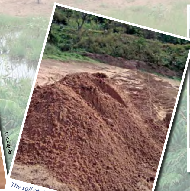
The sludge is covered with soil immediately after offloading on site to prevent possible odours.
