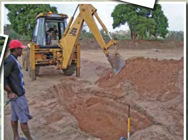
The sludge is covered with soil immediately after offloading on site to prevent possible odours.
