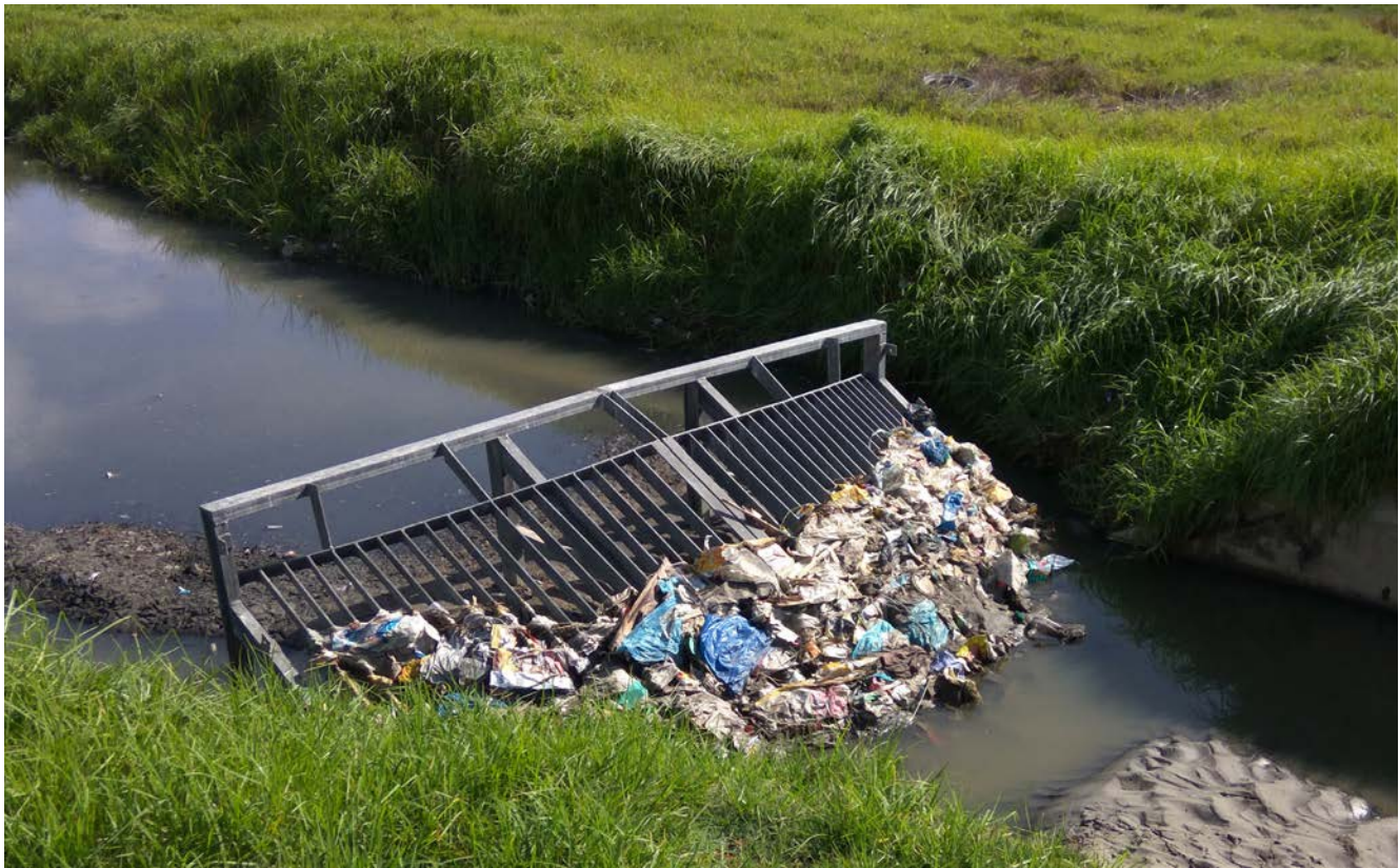
This image from 2019 shows broken 'nightsoil' bags and other waste at a stormwater outlet that discharges into Milnerton Lagoon. The City of Cape Town's Water and Sanitation Directorate installed a larger litter trap in March 2022, and in November created a sandbag barrier to dam up the polluted stormwater, which is then pumped into the sewer line and conveyed to Potsdam WWTW. Litter traps are being installed in stormwater channels upstream, and a low-flow diversion of stormwater into the sewage system is being investigated.
