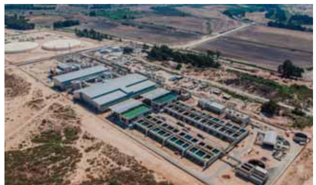
The Sorek desalination plant, 15 km south of Tel Aviv, is the largest in Israel.
