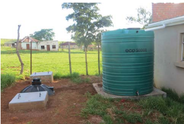
Biodigesters were installed at 14 households that already had water storage tanks and access to cattle nearby, since the biodigesters needed to be 'fed' with water and cow dung at least every five days. Two control digesters with full-gas profiling and meteorological measurement capability were installed at SolarWatt Park on the Alice Campus of the University of Fort Hare.
