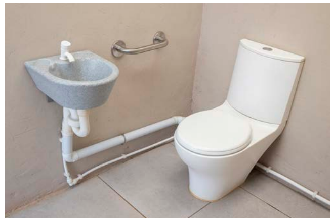
Bakerville Primary School is located in Ngxabaxa Mount Frere, in the Eastern Cape. The school has 172 learners, and had only 3 pit latrines that had deteriorated significantly. The Arumloo low-flush toilet and associated DEWdrop ecological wastewater treatment system presented an opportunity to address the challenge of effective robust sanitation delivery to provide hygienic and dignified school sanitation facilities.
