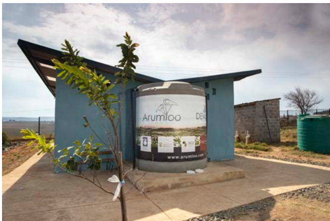
Bakerville Primary School is located in Ngxabaxa Mount Frere, in the Eastern Cape. The school has 172 learners, and had only 3 pit latrines that had deteriorated significantly. The Arumloo low-flush toilet and associated DEWdrop ecological wastewater treatment system presented an opportunity to address the challenge of effective robust sanitation delivery to provide hygienic and dignified school sanitation facilities.
