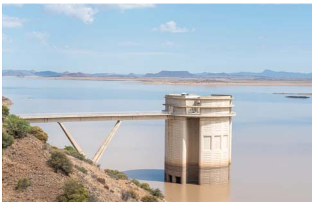
The Orange-Fish tunnel inlet in the Gariiep Dam. One of Dr Meiring du Plessis's first tasks at the Soil and Irrigation Research Institute in the 1960s was to quantify the potential effect of Orange River irrigation water quality on the soil in the Fish River catchment, to which it was to be transferred.
