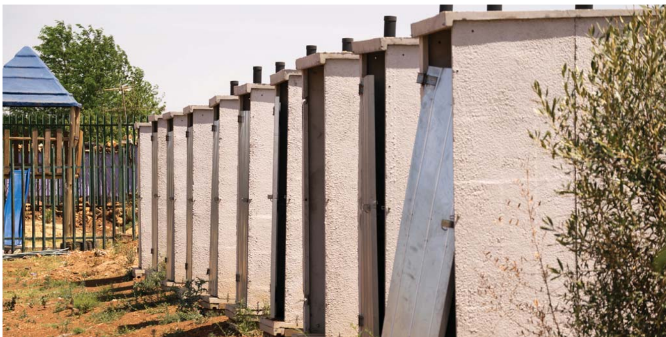
VIP toilets at a primary school. Access to improved sanitation has increased from 61.7% in 2002 to 83.3% in 2023.
