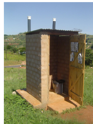
One of the 80 000 urine diversion toilets rolled out by eThekweni Water and Sanitation.
