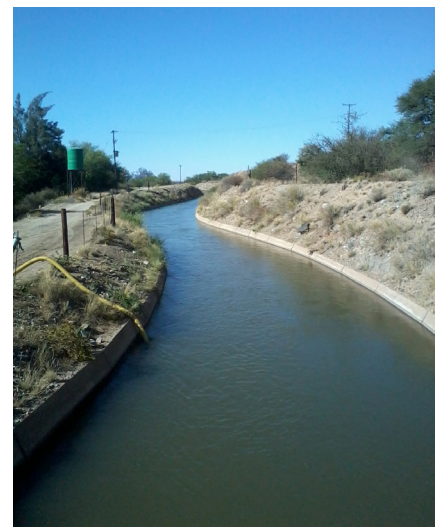
Below: A typical irrigation water canal.
