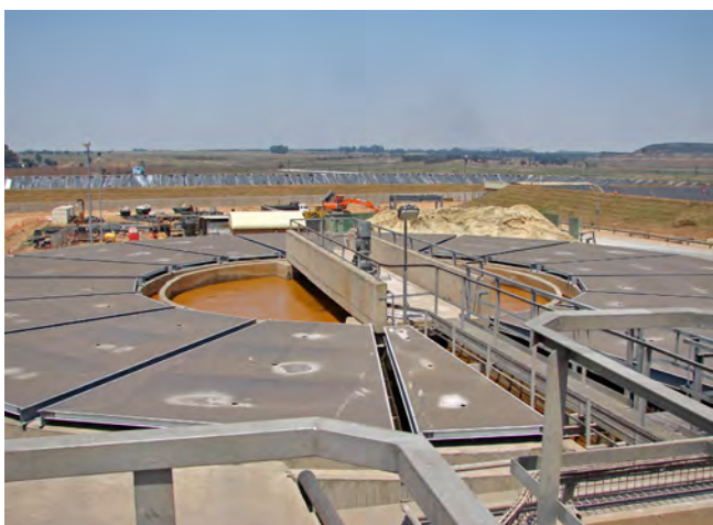
Initiatives such as the award-winning Emalahleni water reclamation plant situated at Witbank, which desalinates mine-water for resale to the Emalahleni Local Municipality, proves that South Africa possesses the know-how to deal with its water challenges. (Credit: Lani van Vuuren)
