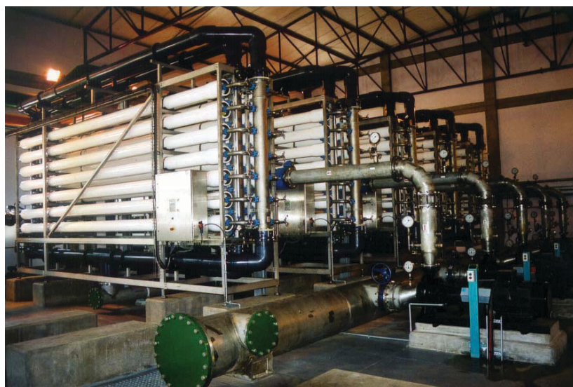
The ultrafiltration unit process, which acts as a final barrier against harmful pathogens
