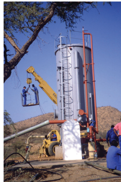
Erecting the carbon filter at one of Windhoek's injection boreholes
