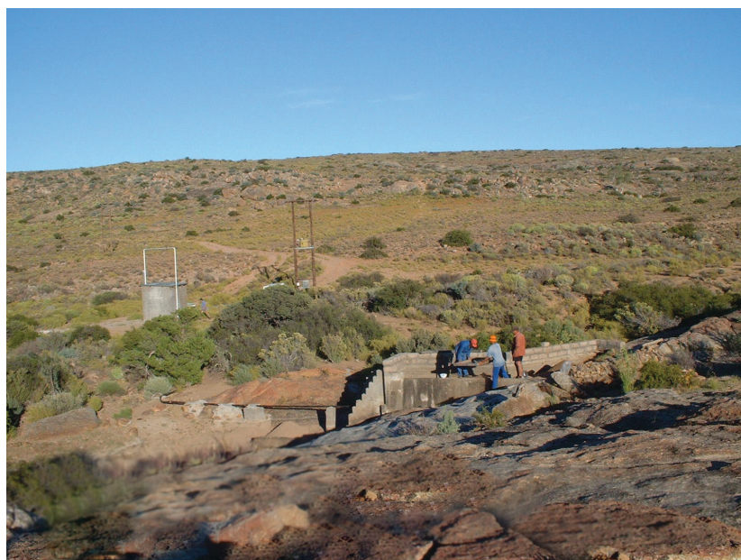
Sieving sand for rehabilitation of the sand filter. In the background is the pump house of the abstraction borehole.
