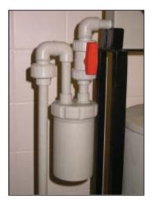
Water flows from a slipstream of the main process water, into the Rotoscope through this pipe, before being channelled up to the rotating plastic wheel.
