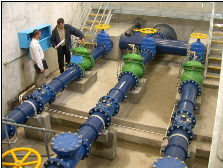
Figure 4 Internal view of a portion of the 1065 mm diameter chamber
