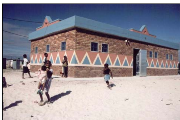
Figure 6 Completed chamber in Khayelitsha
