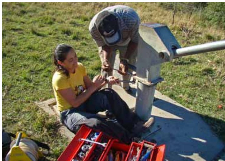
At times simple maintenance rather than complex scientific solutions are required to provide sustainable services. Here CSIR geohydrologist, Sumaiya Clarke, is assisting to repair a handpump.
