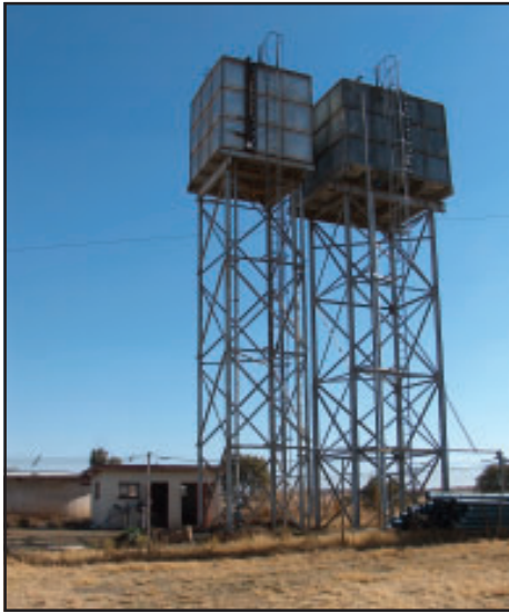
Left: A groundwater storage facility at Dealesville in the Free State – a small town with a water supply scheme based on boreholes.
