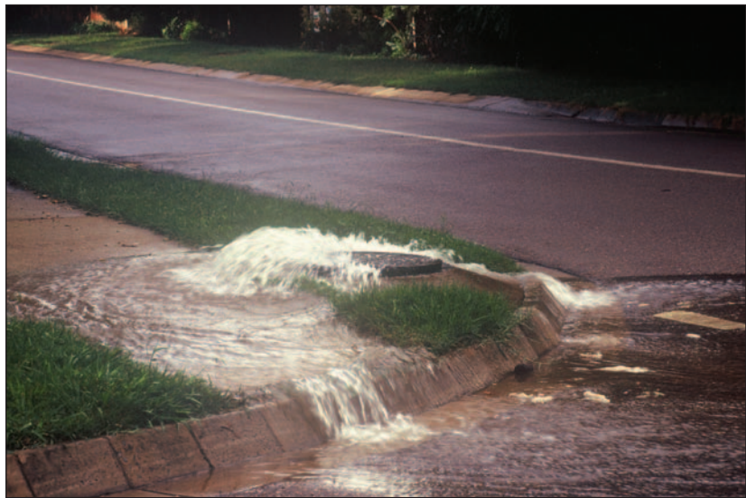
Extraneous flow can reduce the originally designed capacity of a sewage collection system.
