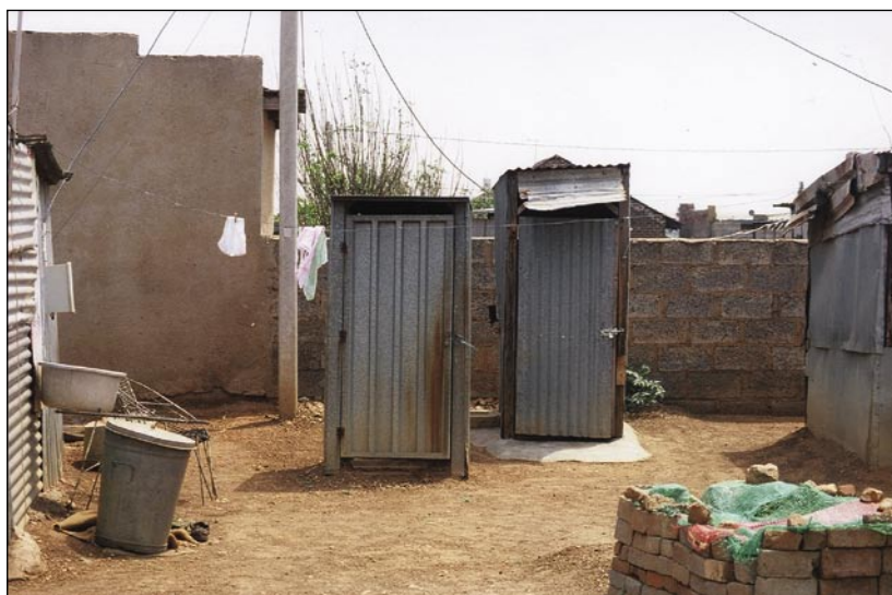
A national audit has found that up to 28% of household sanitation systems (mostly basic sanitation) have failed or are in the process of failing.
