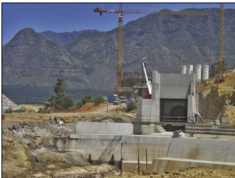
In November the Berg River was closed off by the dam, and diverted temporarily through the outlet conduit shown here.
