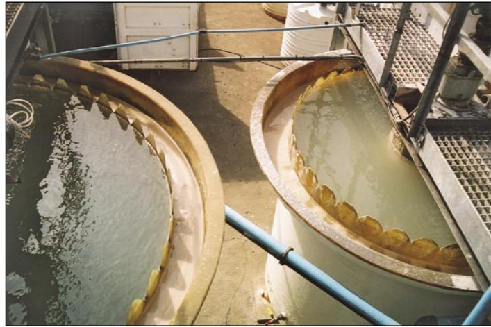
After the pre-treatment process the water is clarified before being sent through the ultrafiltration membranes.
