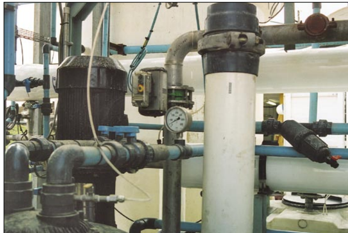
Spiral reverse osmosis (RO) membranes are used to remove salinity in the water. Up to 500 RO membranes will be installed on the main plant.
