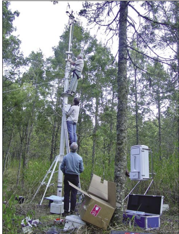
A telescopic mast is used to install the equipment high enough above the Podocarpus falcatus canopy at Tzaneen. Here project team members Drs Colin Everson, Caren Jarman and Peter Dye can be seen in action, mounting sensors to the mast.
