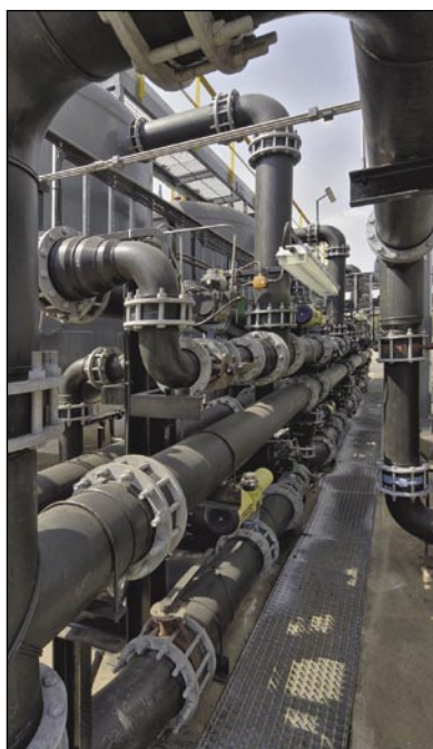
Process water is treated at a rate of up to 2 000 m 3 /h and is then reused.
