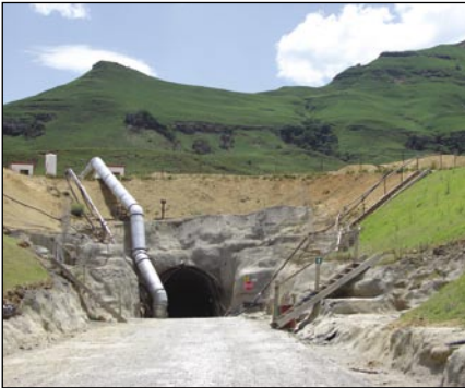
Entrance to the 5 m x 5 m exploration tunnel. The 6 m 3 dump trucks used at present will later make way for articulated dump trucks once construction of the main machine hall starts. Passing bays are being excavated every 100 m along the tunnel to permit empty trucks give way to fully laden trucks hauling uphill.
