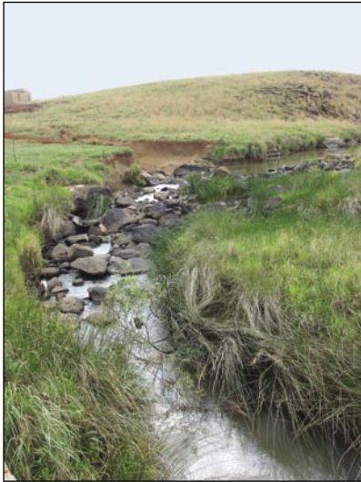
The Braamhoek Spruit will be dammed by a roller-compacted concrete wall. Compensation flows will, however, ensure uninterrupted flow to downstream users.
