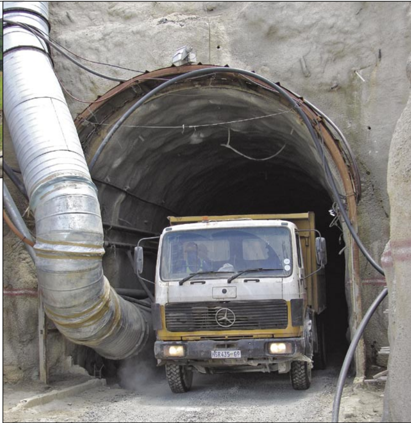
Entrance to the 5 m x 5 m exploration tunnel. The 6 m 3 dump trucks used at present will later make way for articulated dump trucks once construction of the main machine hall starts. Passing bays are being excavated every 100 m along the tunnel to permit empty trucks give way to fully laden trucks hauling uphill.
