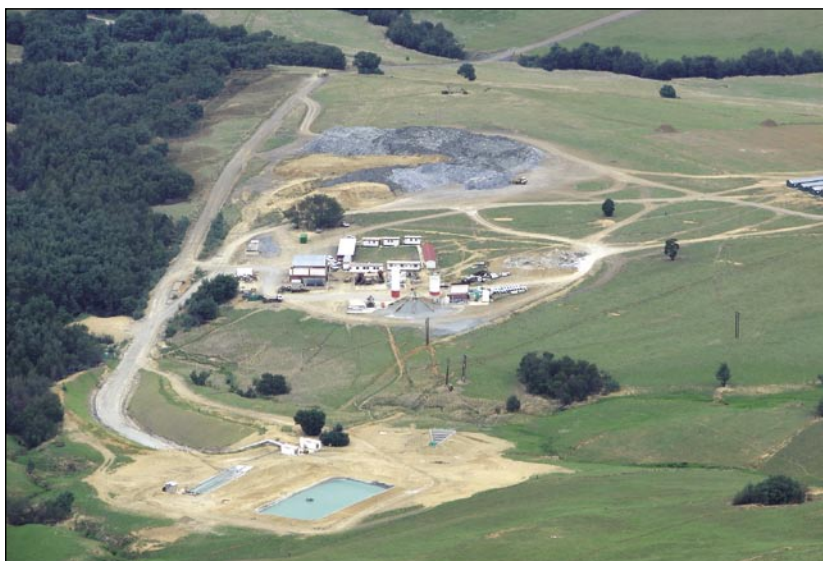
An aerial view of the present construction site. The entrance to the exploration tunnel is on the left. Unlike the Drakensberg Pumped Storage Scheme, no permanent construction village is planned for the site.
