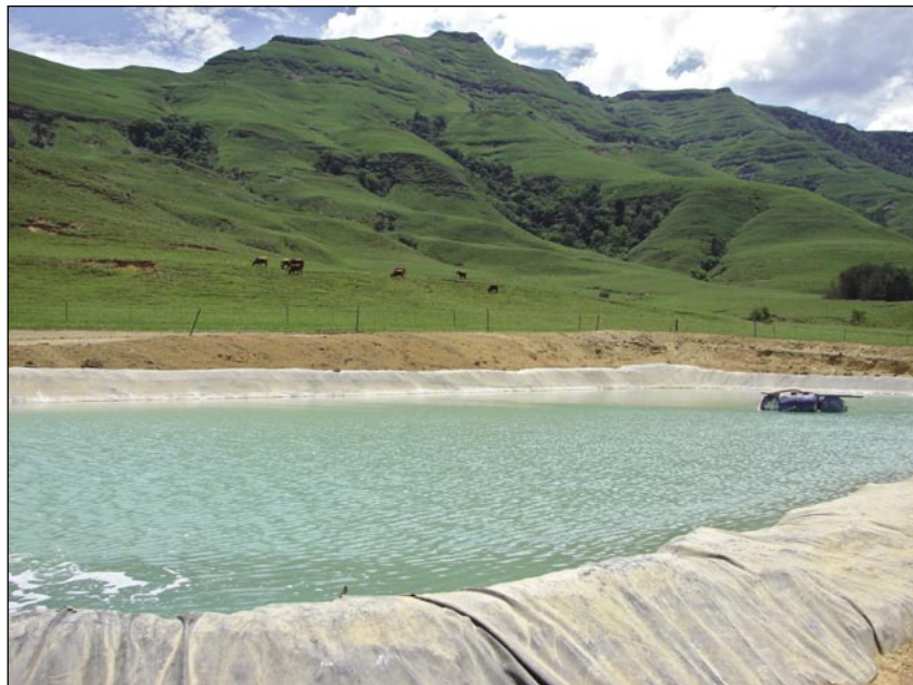
All water from the tunnel is pumped to a holding dam before being treated and released back into the river system. Solid waste is also strictly controlled.
