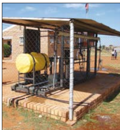
The 10 000 ℓ membrane plant erected at Madibogo Bathlaping Primary School to test the applicability of this technology for rural applications.
