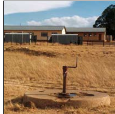
Poorly sited borehole near a school pit latrine.
