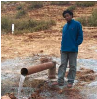
Artesian borehole at Makhoba near Matatiele.
