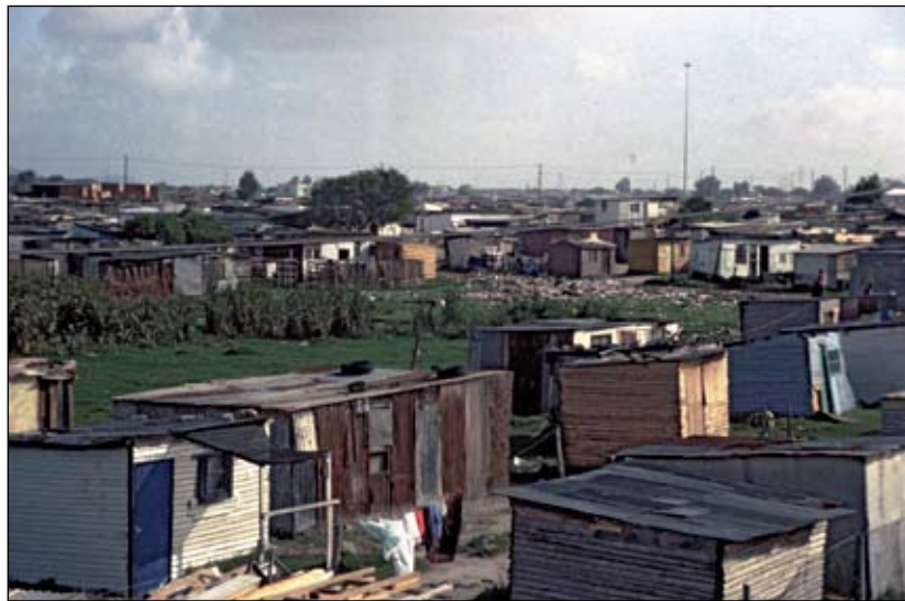
Water, sanitation and hygiene are essential underpinnings to home-care strategies.
