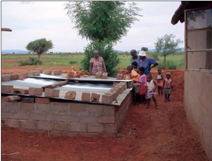
An example of a closed reservoir used to store rainwater for food growing purposes.
