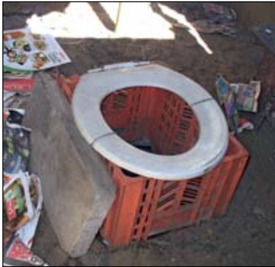
In many cases the toilet structures assessed bore ample opportunity to cause or transmit disease.
