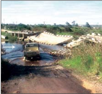
This bridge in the town of Heidelberg, Western Cape, failed as the foundations were undermined. The fact that piers on the upstream side failed suggests that local scour was responsible.
