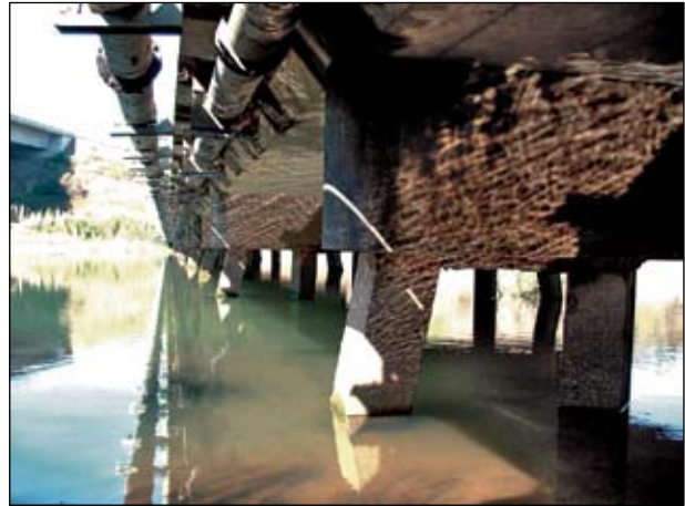
The piles of this bridge near the Mzimkulu River mouth have been exposed to a significant depth.
