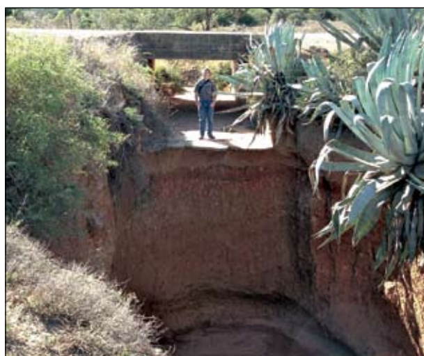
Constriction of the flow at this culvert near Riebeeck East, northwest of Grahamstown, in the Eastern Cape, has led to high velocity water exiting the downstream end. The riverbed has been severely scoured for a long distance downstream.
