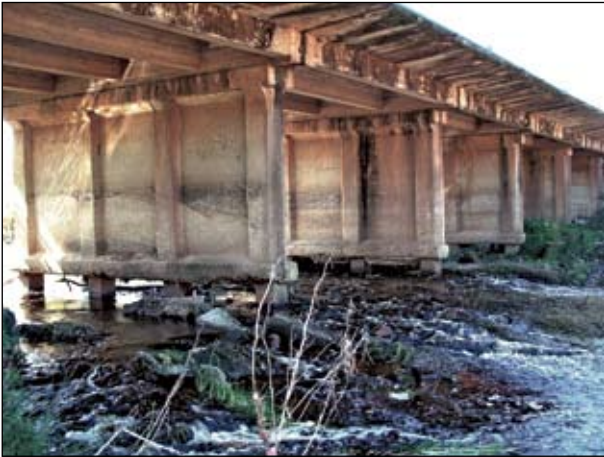
The Palmiet River in the main stream of Grabouw, in the Western Cape, no longer flows parallel to the bridge piers. This may have initiated scouring under the bridge and exposure of the piles.
