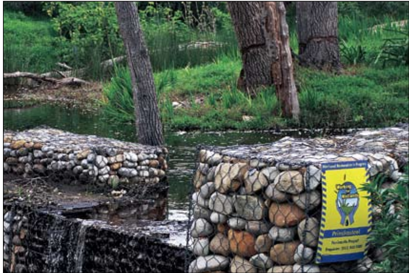
Higher in the catchment, restoration of the Prinskaasteel River is being conducted as a Working for Wetlands project. Gabions have been built to arrest erosion that was resulting in loss of wetland habitat.
