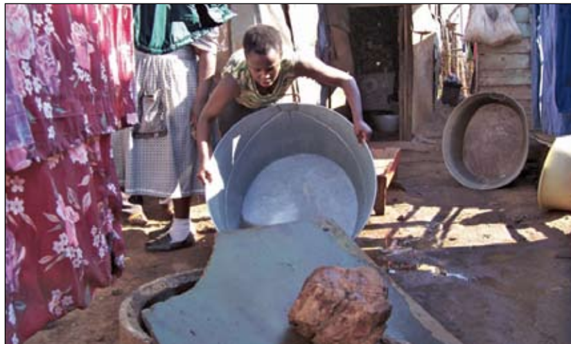
Greywater disposal down a stormwater manhole.
