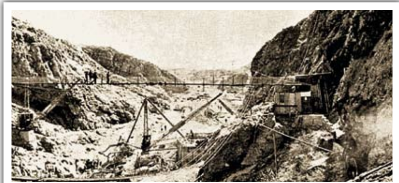
Cable way at Hartbeespoort Dam during the construction of the foundations, 1922.
