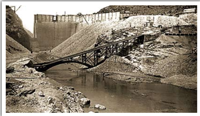
Hartbeespoort Dam during construction of the wall.
